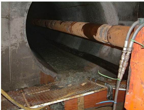
Figure 2-1 Boring of a horizontal deposition hole (KBS-3H).
