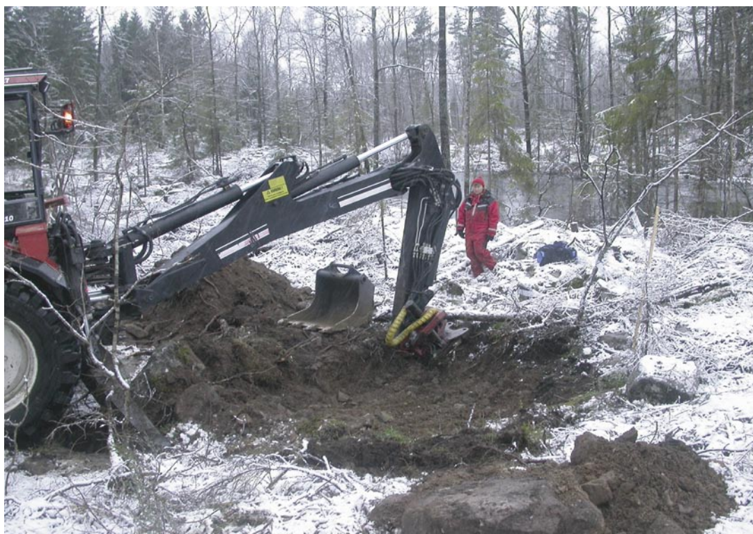
Figure 3-1. Kärstin Malmberg Persson and tractor-excavator.
