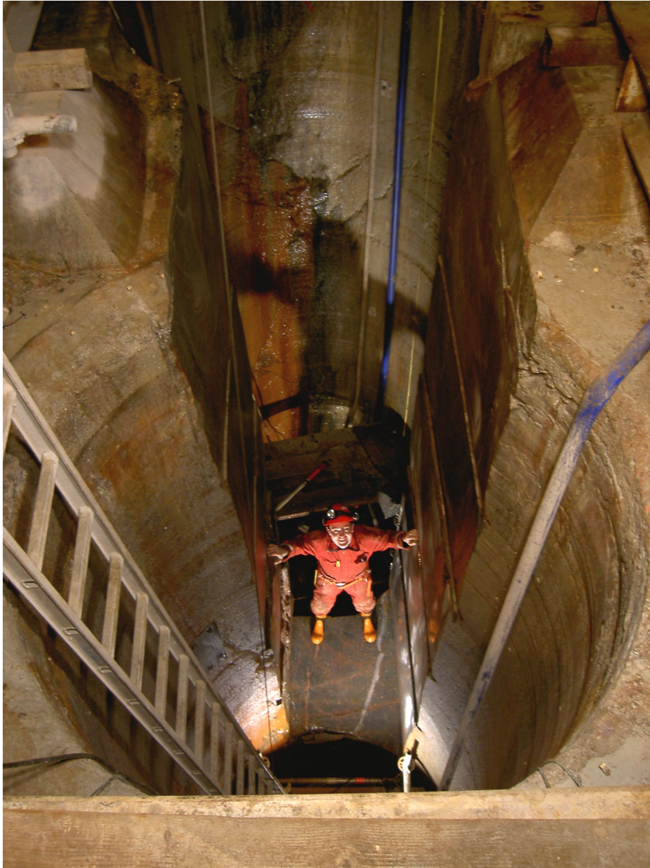
Figure 3-4 Photograph of the experiment site after removal of the five one metre high pillar blocks between the two large holes.
