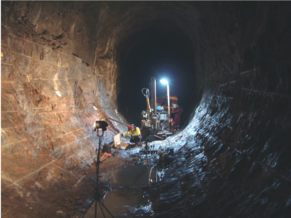
Figure 3-2 The Apse experimental drift shortly after the excavation.
