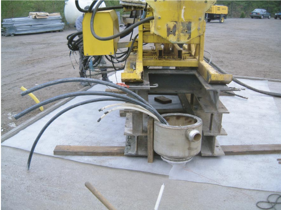
Figure 5-9. The water discharge header and hoses for air-lift pumping.
