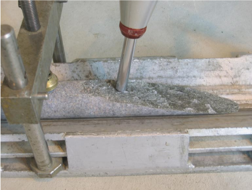
Figure 3-2. Clamp for the Schmidt hammer tests.
