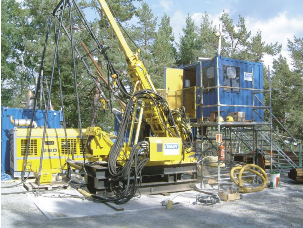
Figure 4-2. The KSH03 drill site.
