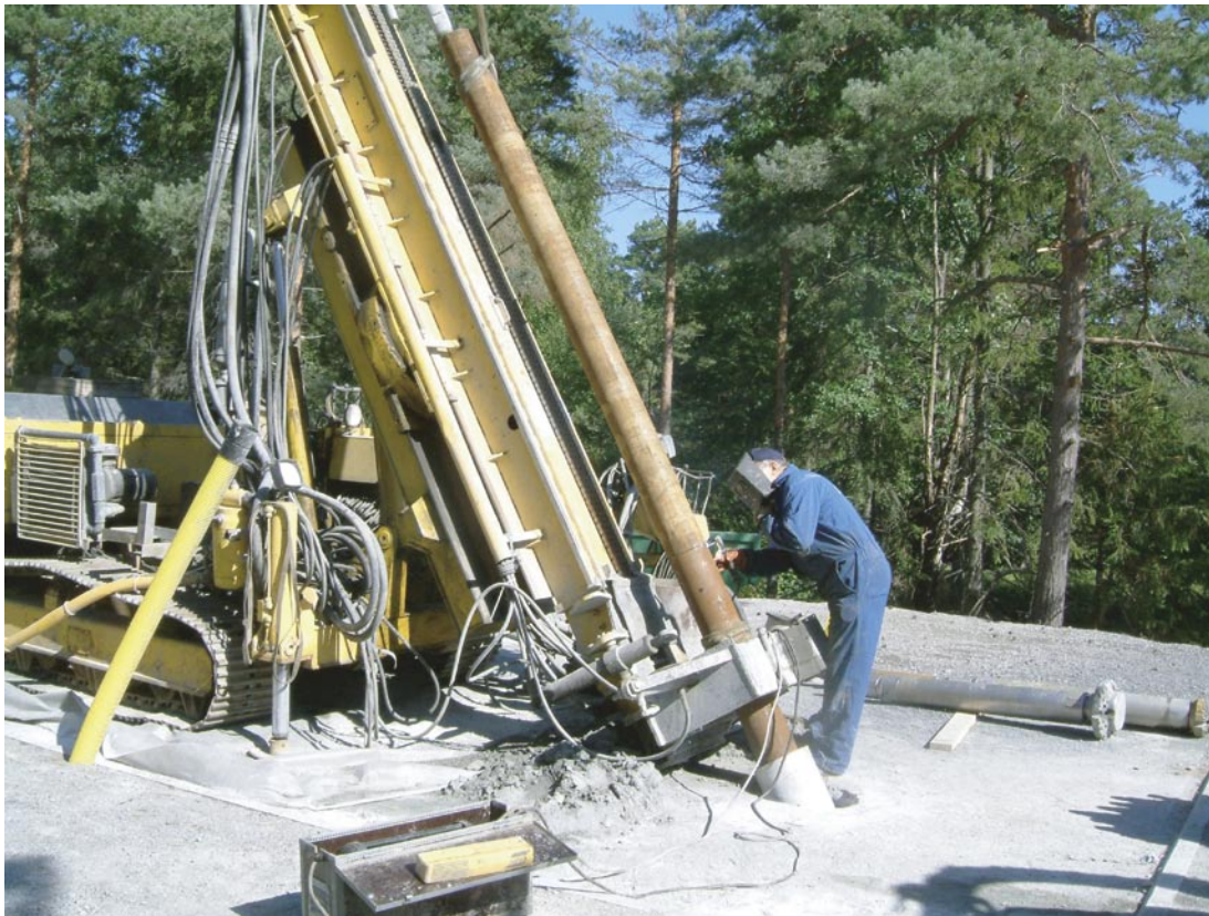
Figure 4-1. Percussion drilling equipment.
