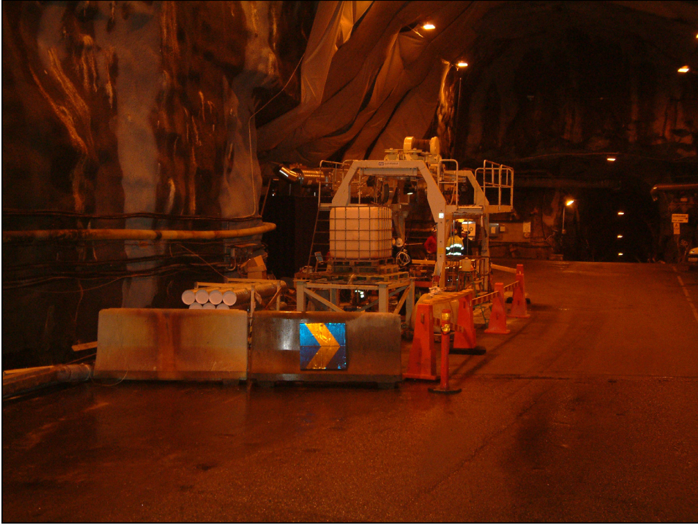
Figure 3-21. The TBM assembly hall/ the Lasgit site
