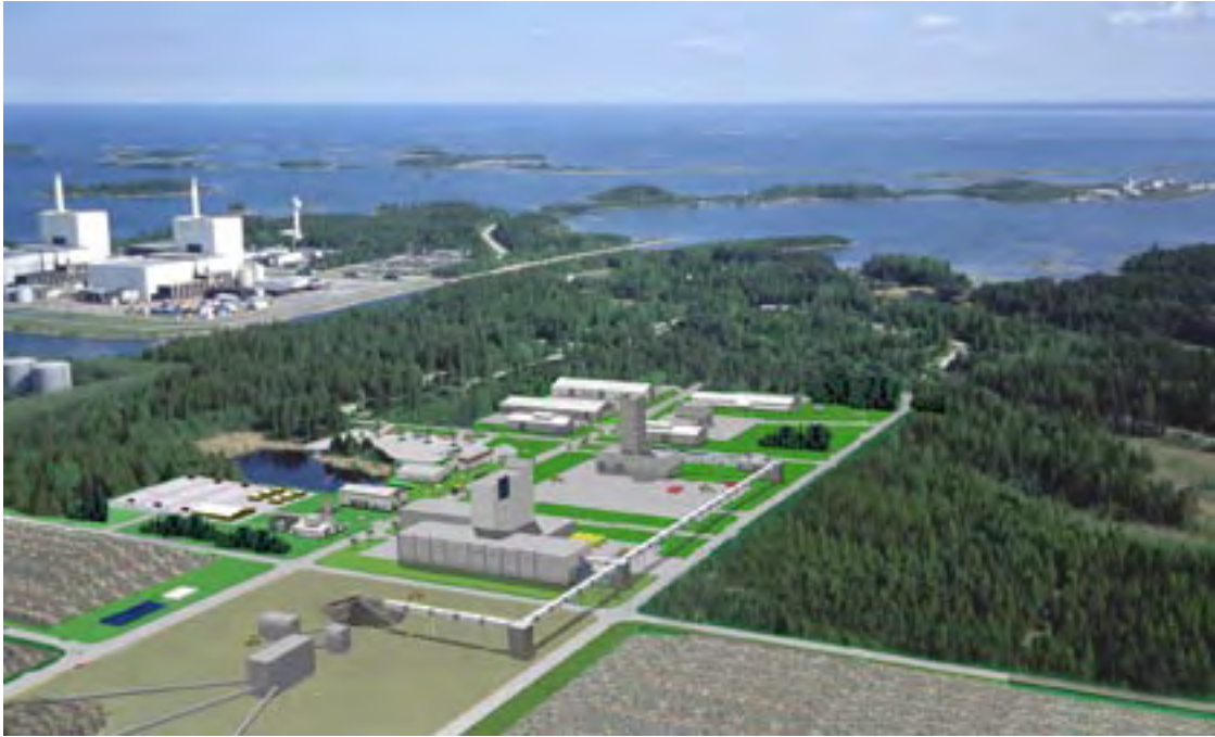
Figure 11-3. Deep repository operating area at the entrance to the Forsmark nuclear power plant during the Layout D0 step.
