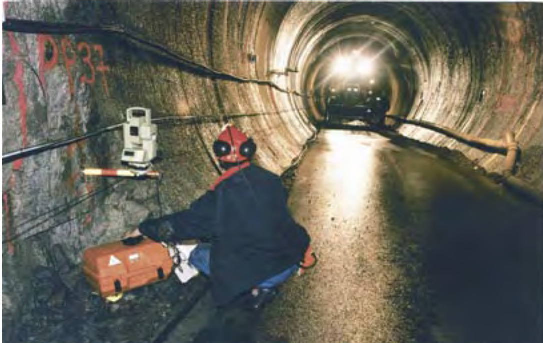
Figure 1-2. The Äspö HRL consists of a 3,600 metre long tunnel that goes down to a depth of 460 metres.
