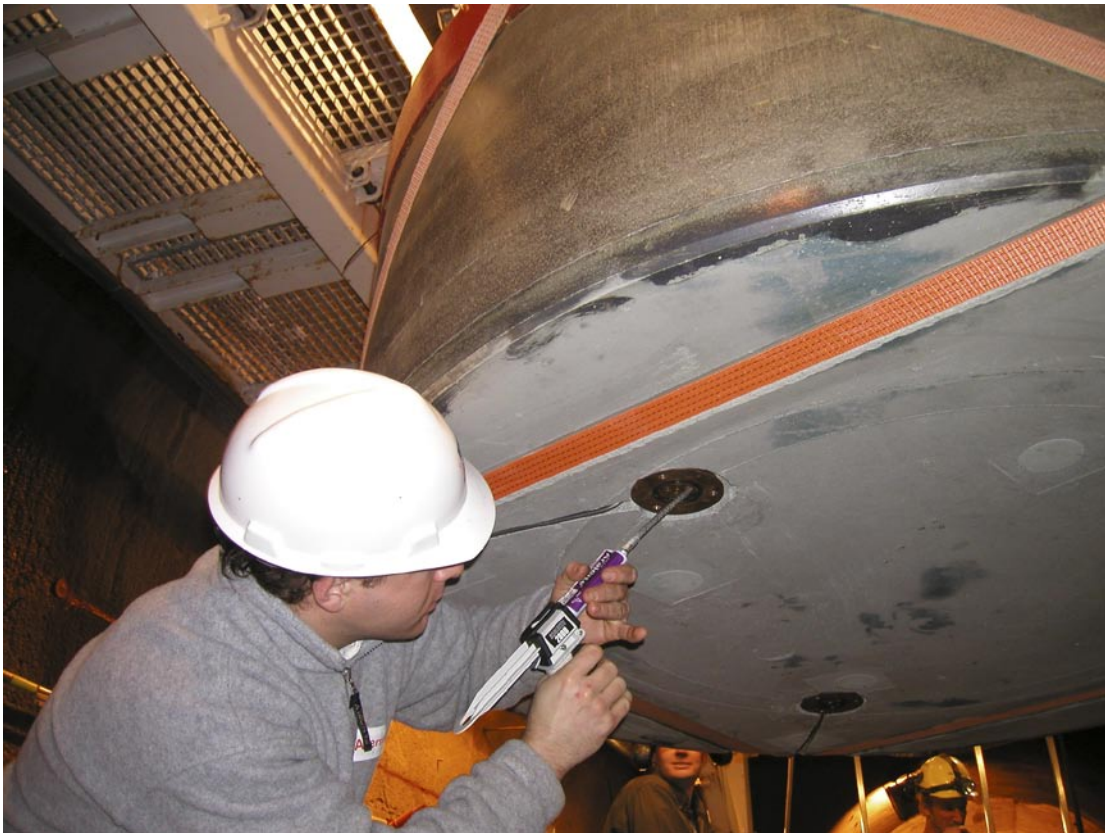
Figure 6-11. Photos showing the installation of vertical displacement sensors.
