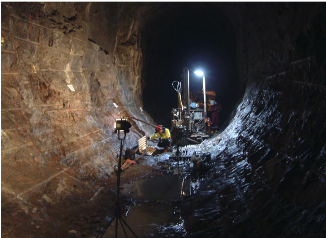
Figure 3-2. The experimental TASQ tunnel shortly after the excavation.
