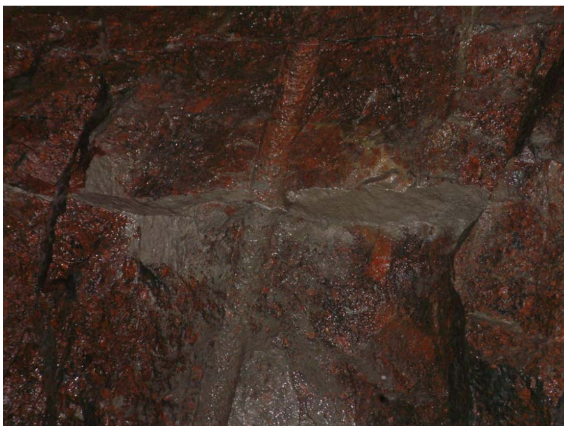
Figure 5. Evidence of grout penetration (sometimes on two sets) and joint deformation due to pre-grouting pressures.
