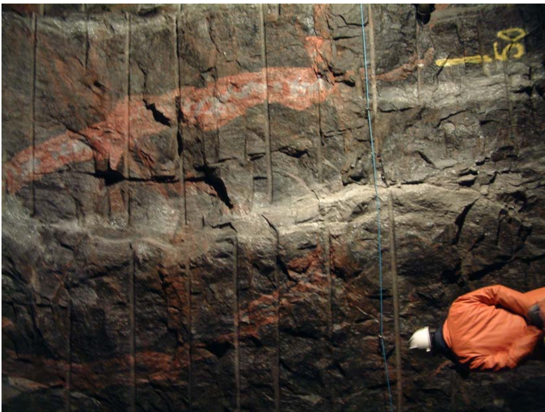
Figure 4. Excellent quality and numerous half-rounds in walls (both) and arch are evident between ch. 47 to 53m, probably due to reduced jointing.
