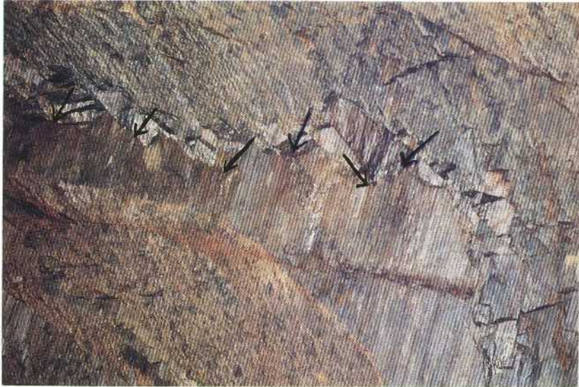
Several point leakages from a fissure en echelon, in the contact leptite - amphibolite. 4/258
