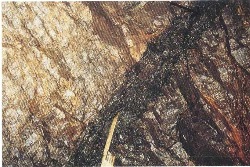
Point leakage (v) from thin amphibolite plate parallell to the schistosity. The amphibolite is partly altered to clay and surrounded by granite gneiss. 0/785
