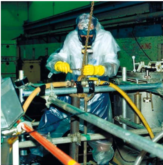
Figure 8-4. Preparation work prior to plant dismantling operations.
