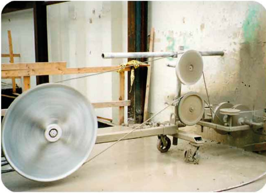
Figure 7-11. Typical Wire Saw drive in action cutting a section of wall.
