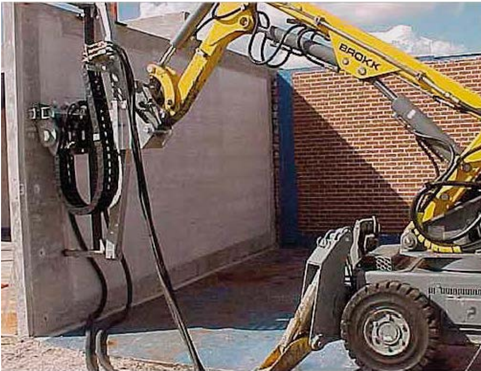
Figure 7-10. Floor Shaver mounted on a machine for wall decontamination.
