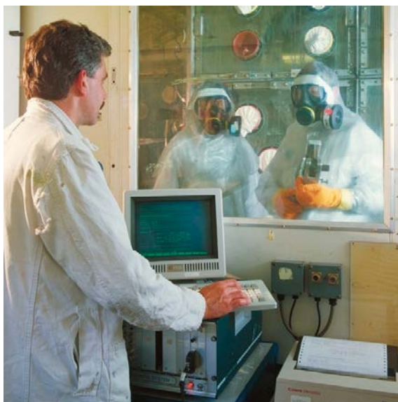
Figure 8-2. Manual dismantling operations utilizing Re-usable Modular Containment (RMC).
