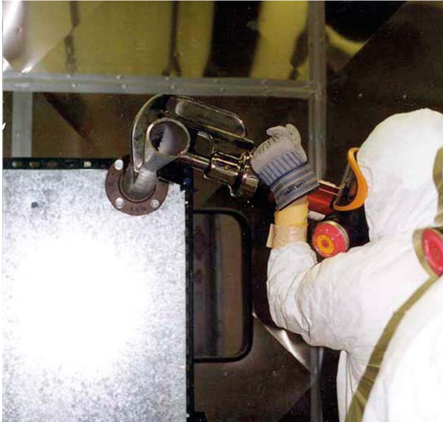
Figure 7-6. Blade Plunging Cutter being used to cut 2.5 inch OD pipe.
