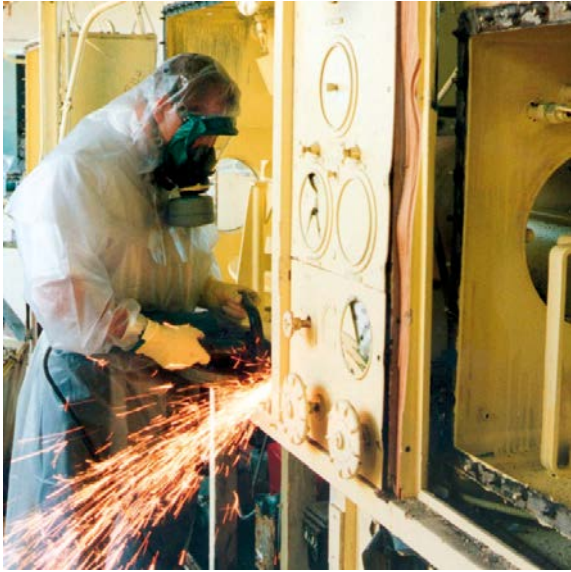
Figure 8-5. Typical manual plant dismantling operations.
