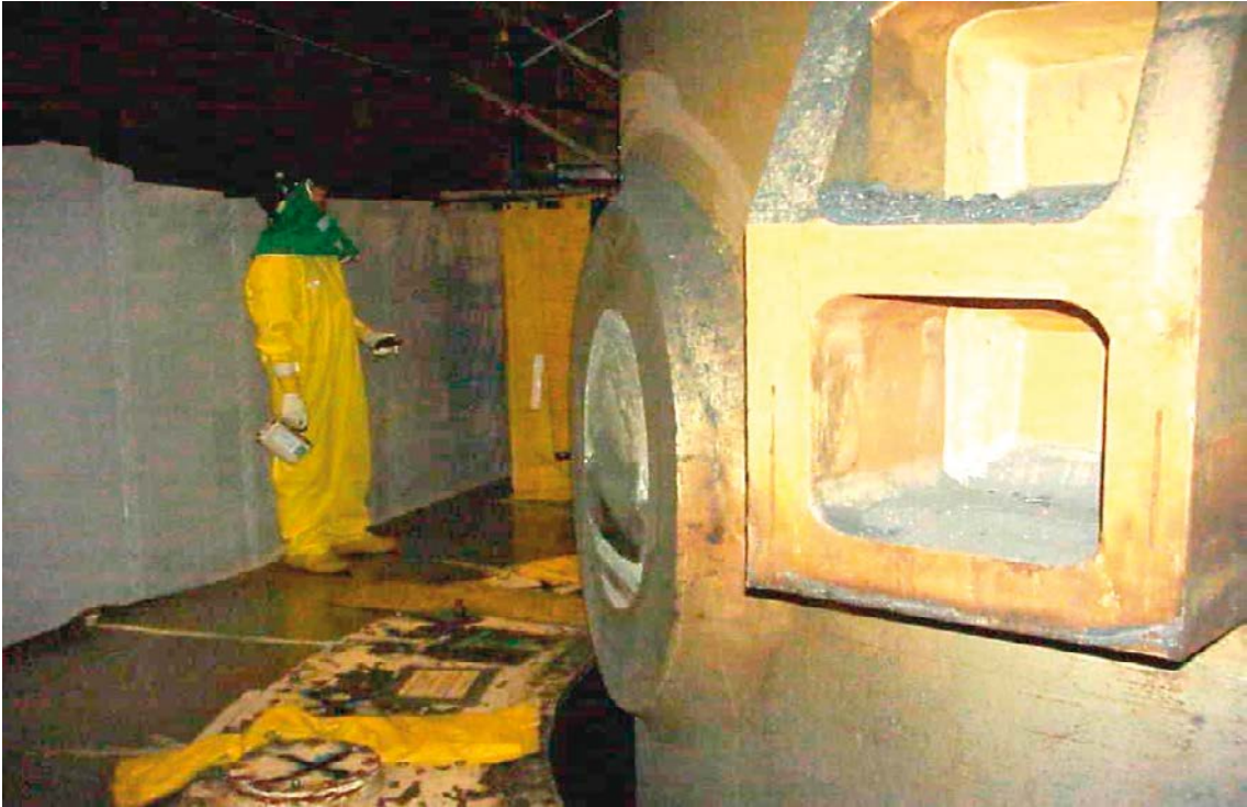
Figure 7-3. San Onofre Unit 1 Reactor Vessel Nozzles after cutting with a diamond wire saw.
