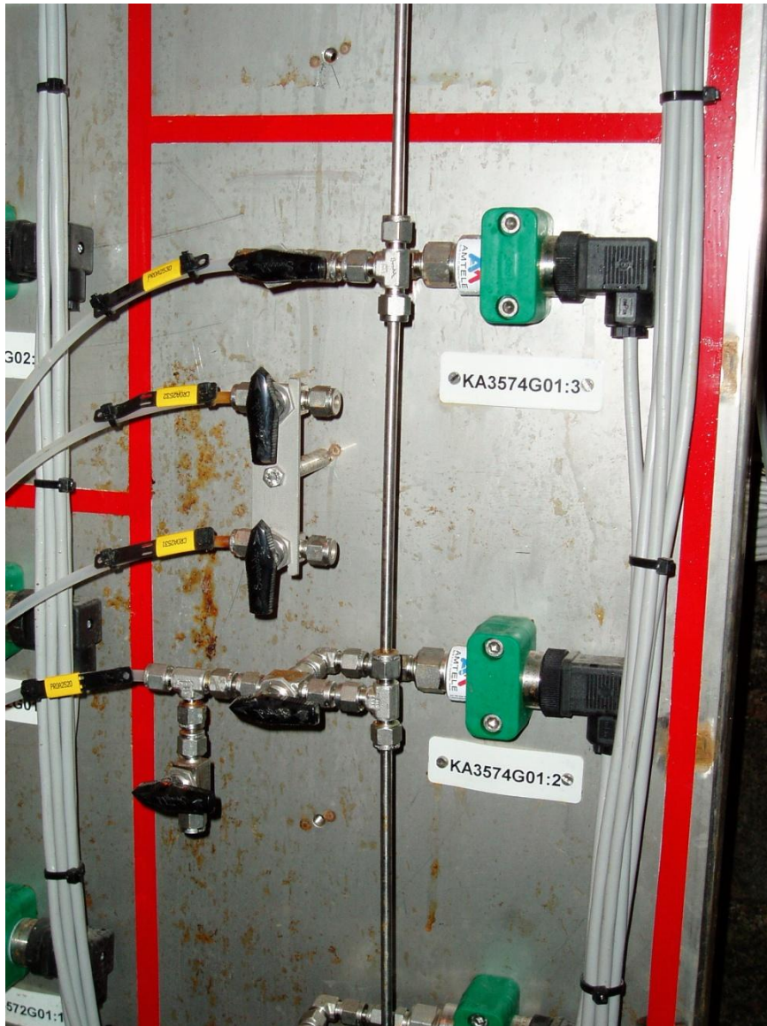
Figure 4-2 Pressure transducers connections
