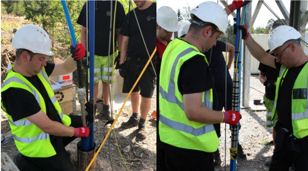
Figure 3-4 Left: Deployment of the downhole termination of the helical cable inside the bullnose (photo: HydroResearch). Right: Fastening of the lowest geophone using heavy-duty cable ties and tape (photo: Sanna Andrén, SKB).
