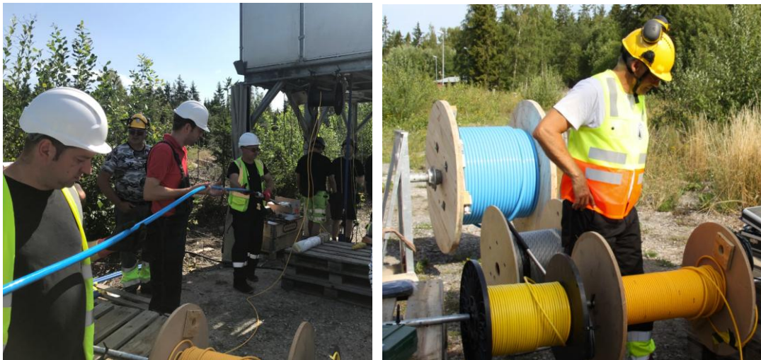
Figure 3-2 Left: Installation in HFM42 using a two-stage podium (photo: HydroResearch). Right: Drums with fibre optic cables (blue, helical and grey, linear) and cables for geophones placed on cable drum jacks (photo: Sanna Andrén, SKB).
