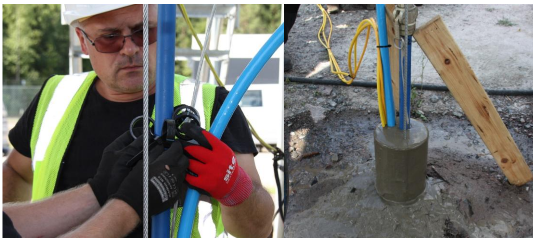
Figure 3-5 Left: Centralizer attached to the grouting pipe (photo: Sanna Andrén). Right: Cement mix has reached TOC, meaning that the entire borehole was filled (photo: Sanna Andrén).
