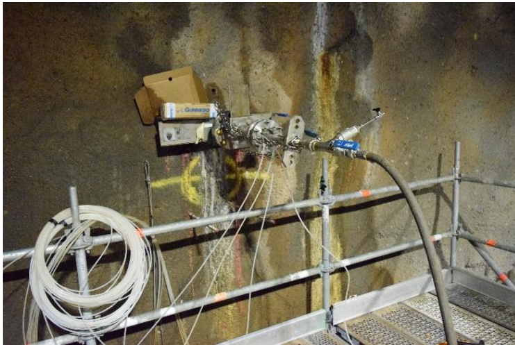
Figure A6-2. Borehole collar K08028F01
