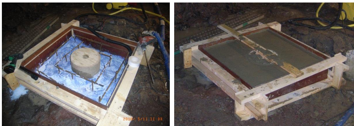
Figure 2-7. Casting of a concrete base.
