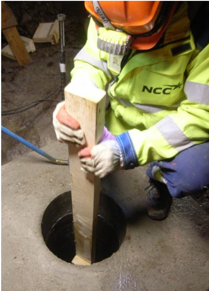
Figure 2-8. Levelling the bottom and measuring the depth of the installation hole.
