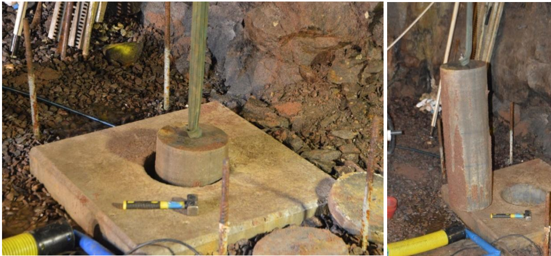
Figure 4-3. The concrete cylinder is being hoisted up from the installation hole.
