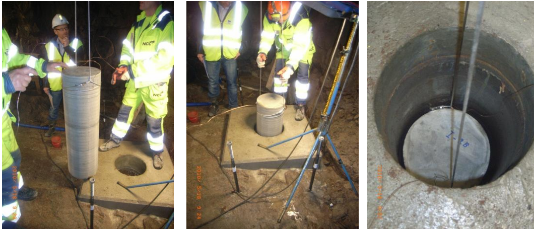
Figure 3-4. Installation of a concrete cylinder.
