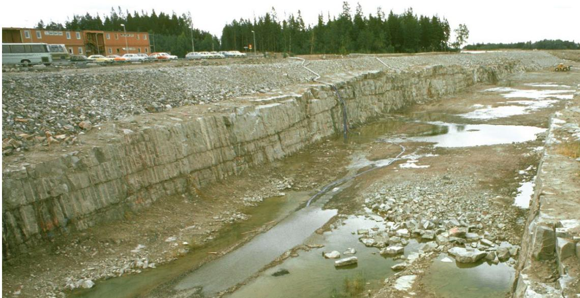
**Figure 7-2.** Picture from the construction of the 13 m deep and more than one kilometre long canal between the Baltic Sea and the nuclear power plant. Horizontal fractures/sheet joints were encountered along the entire excavation. As seen in the picture, there are several “beds” of extensive sheet joints on top of each other. The picture is taken from the southern side of the canal where the current bridge crosses the canal between HFM20 and HFM22 (Carlsson and Christiansson 2007).
