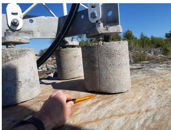
**Figure 4-1.** A possible cause of seasonal variations in baseline results may be temperature-related expansion in one or more parts of the truss mast. Special attention should be given the three anchor points of the truss mast. A slight difference of 0.1 mm due to thermal expansion in one of the anchor points will result in a horizontal motion at the 1-millimeter level in the top of the mast, at the location of the antenna.
