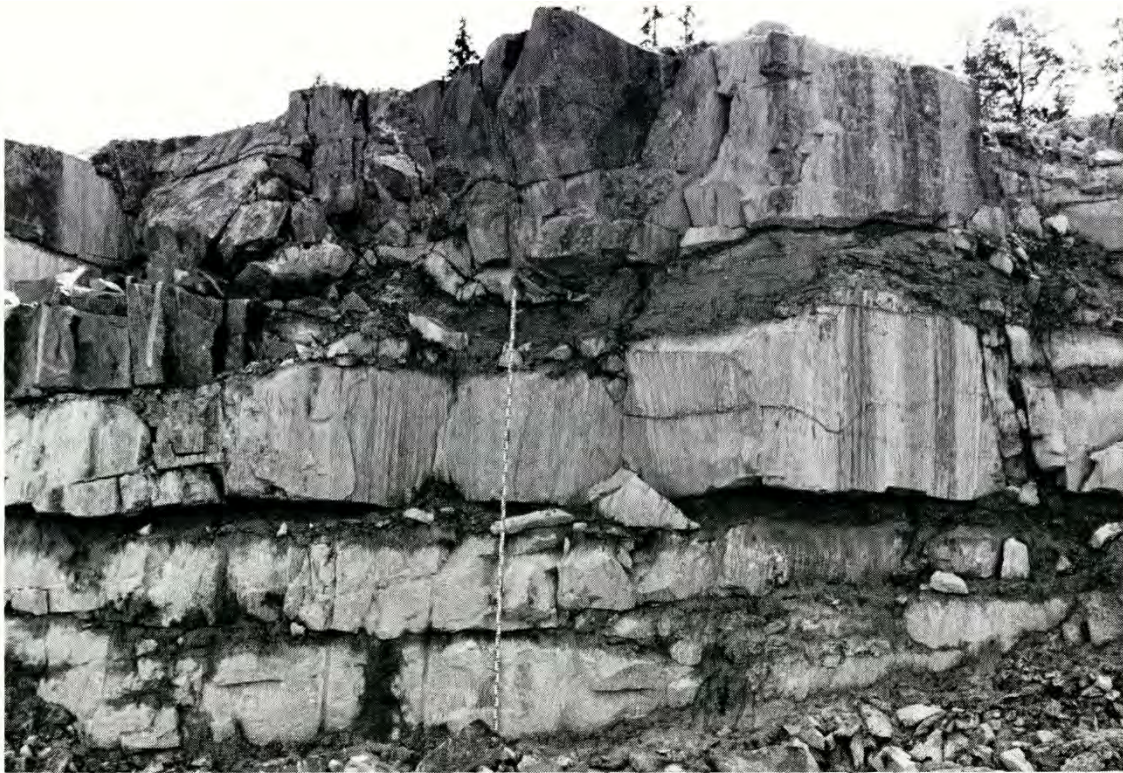
Figure 4-17. Shaft wall along the inlet channel with several sediment-filled sheet joints. The uppermost joint has a maximum aperture of 820 mm. Length of the levelling staff is 4 m. From Carlsson (1979). Photography by G. Hansson.
