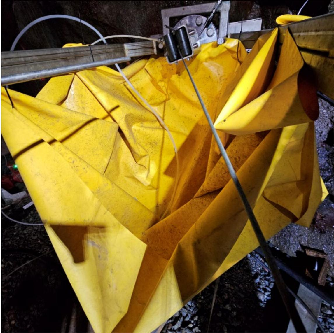
**Figure 4-2** Tarpaulin gathering water that leaks from the borehole sealing mechanism.
