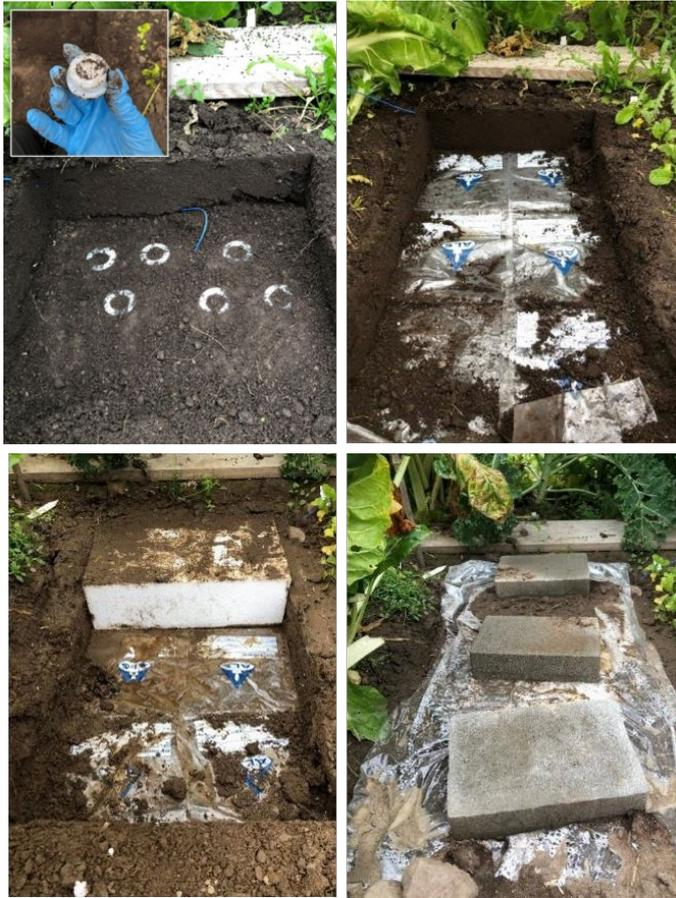
*Figure 5-10. Installation of the DGT devices.*
