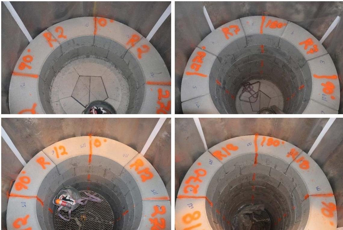
*Figure 5-2. Installation of ring-shaped layers. Top left R2, Top right R7, Lower left R12, lower right R18.*
