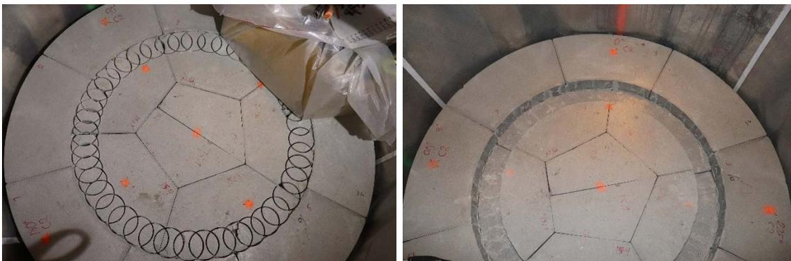
*Figure 4-4. Left: Core drilling of slot in layer C2. Right: Finished slot.*
