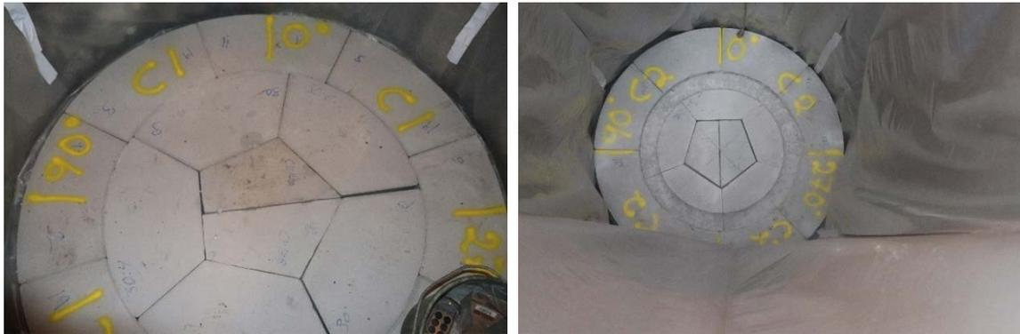
**Figure 5-1.** Installation of bottom layers. Left: layer C1, right: layer C2 with core drilled slot for the canister flange.
