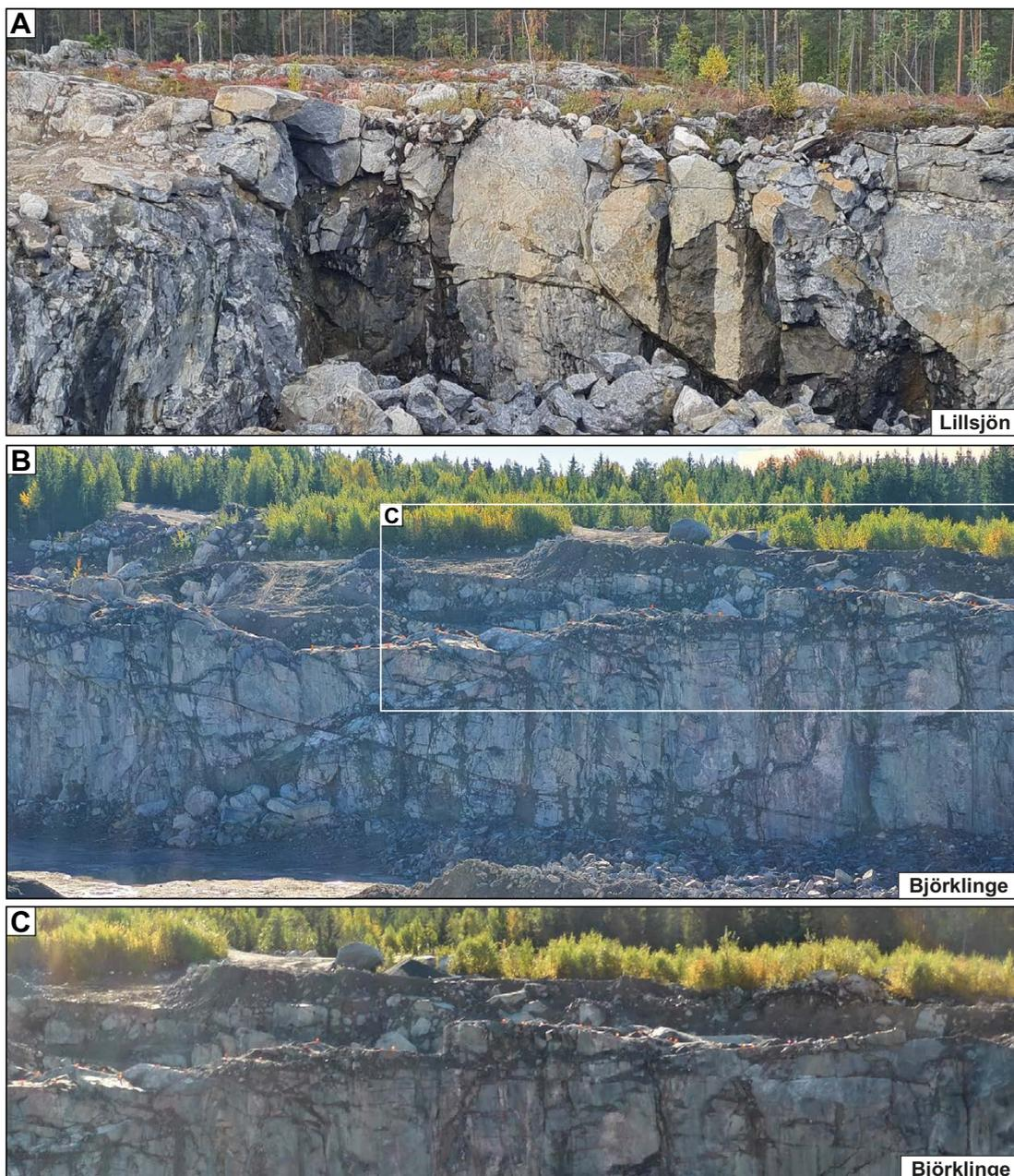
**Figure 4-4.** A. Lillsjön quarry. Gently dipping fractures, with locally dilated fractures in upper 2 m. B. Björklinge quarry with gently dipping and vertical fractures, dilated in the upper part, with fills of diamicton. C. Detail of dilated fractures in upper c. 3 m.
