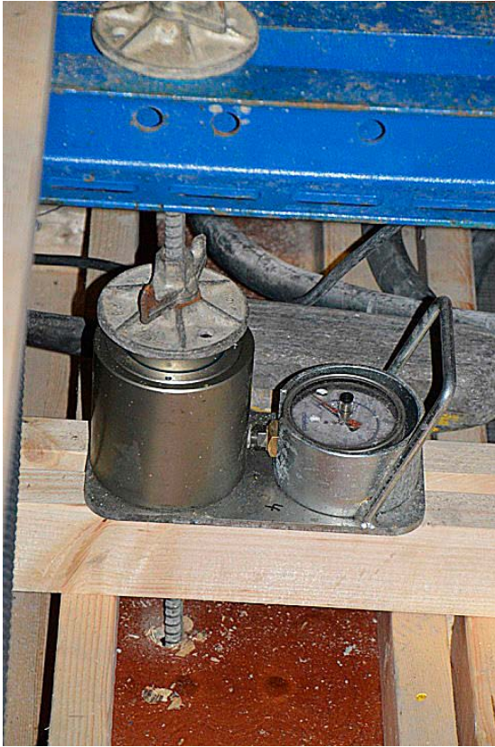
Figure 3-9. Load cell for control of formwork pressure during casting.
