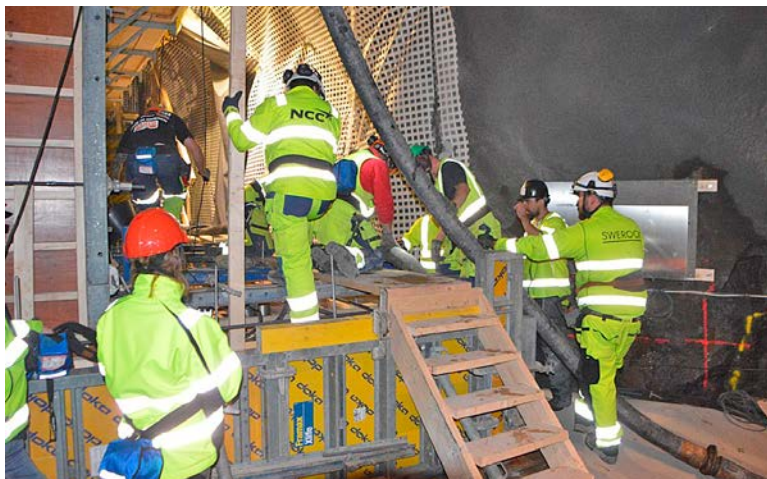
Figure 5-9. Casting of the base slab.
