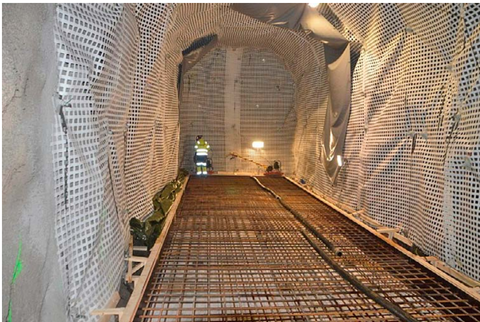
Figure 4-2. All preparations have been made for casting of the concrete slab.
