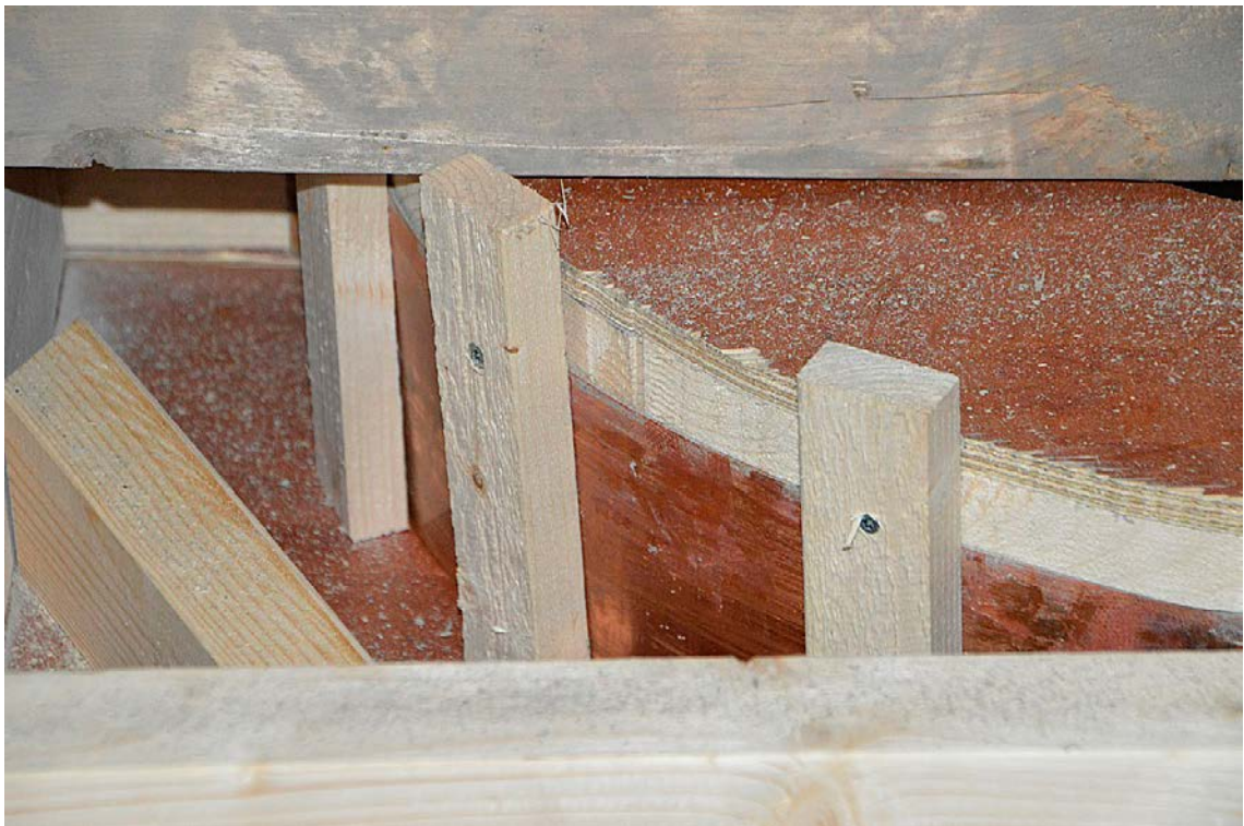
Figure 5-6. A copper joint seal is mounted in the radius between the two walls of section 1.
