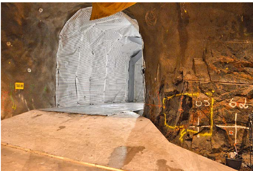
Figure 4-5. All is ready for erecting the formwork for section 1.
