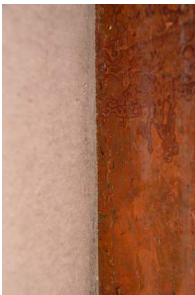
Figure 6-8. Image showing the interface between the concrete and the joint seal.
