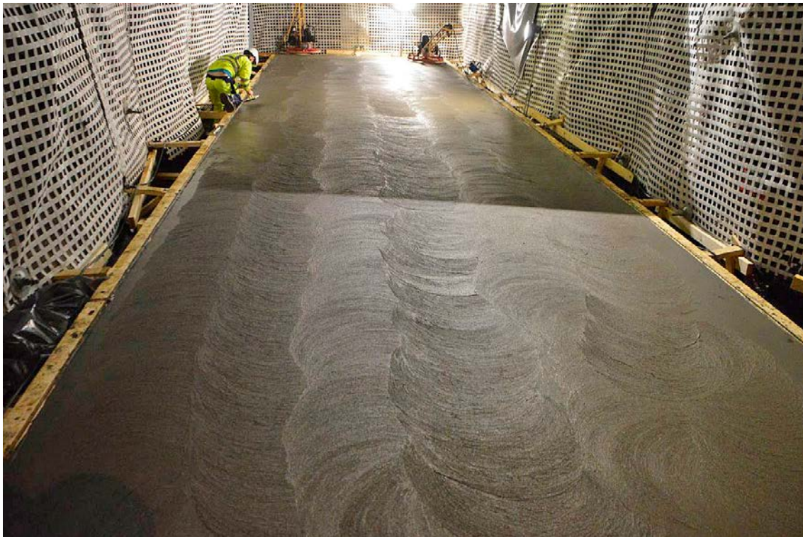
Figure 2-2. Levelling of TAS05 with a reinforced slab on the crushed rock.
