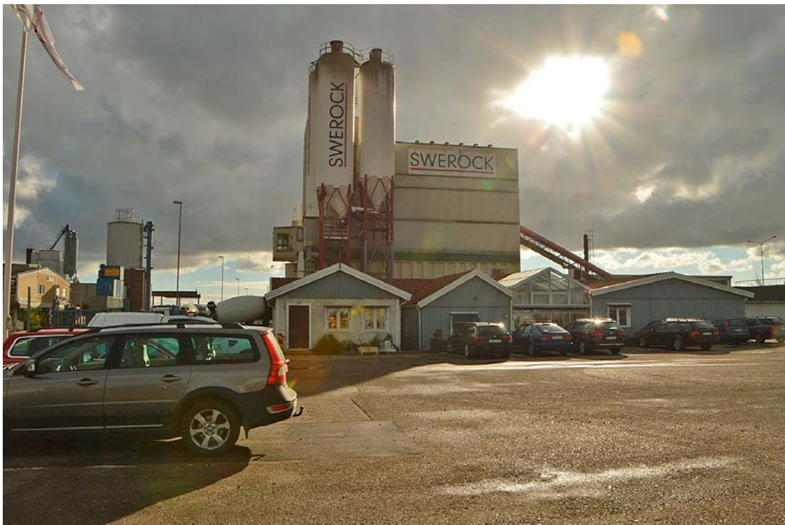
Figure 5-7. Swerock concrete production plant in Kalmar which was used for mixing of the concrete.
