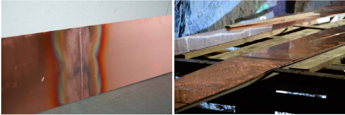
Figure 5-5. Welded copper sheets.
