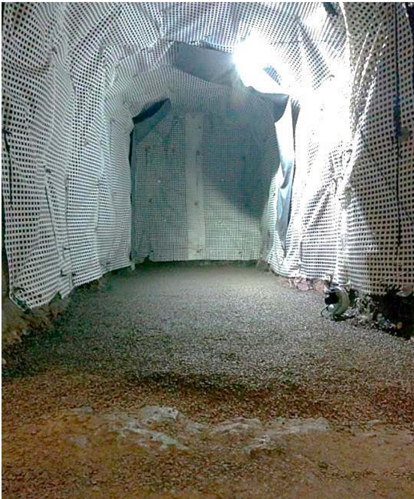
Figure 4-1. TAS05 after rock reinforcement and levelling of the tunnel floor.
