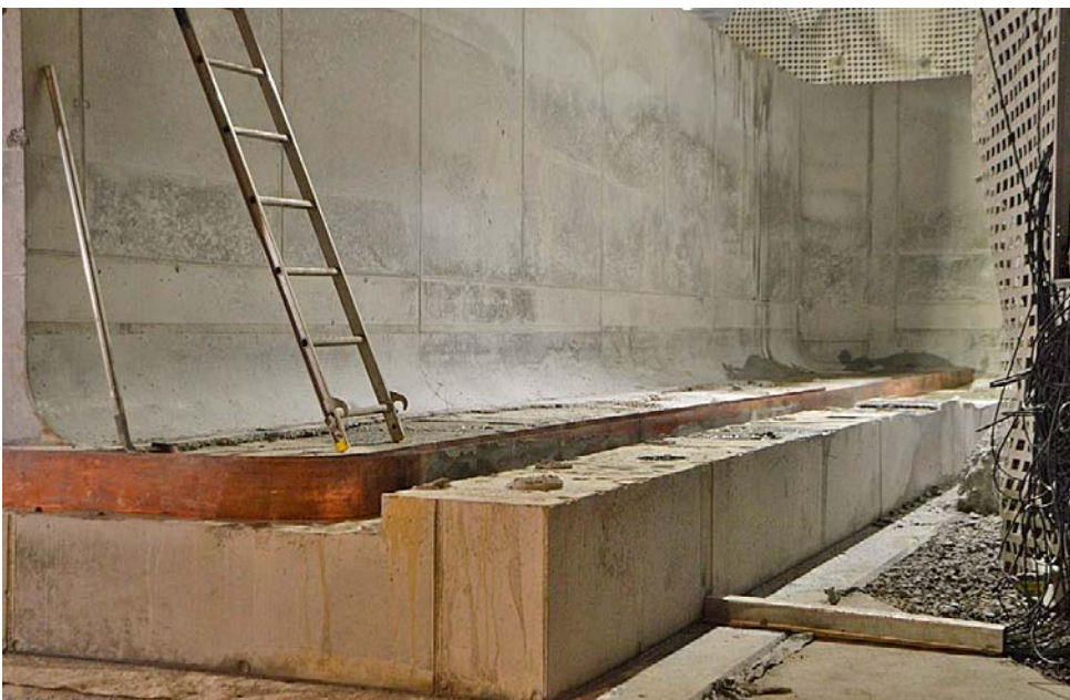
Figure 5-11. Section 1 just after disassembling of the formwork.
