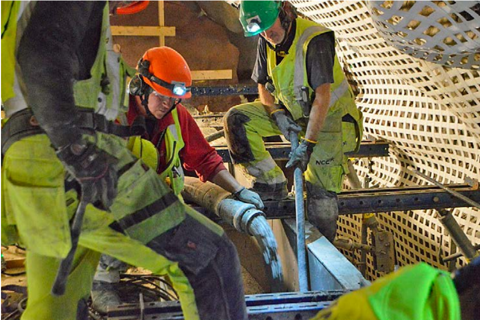
Figure 5-10. Casting of the walls of section 1 and vibrating the concrete.
