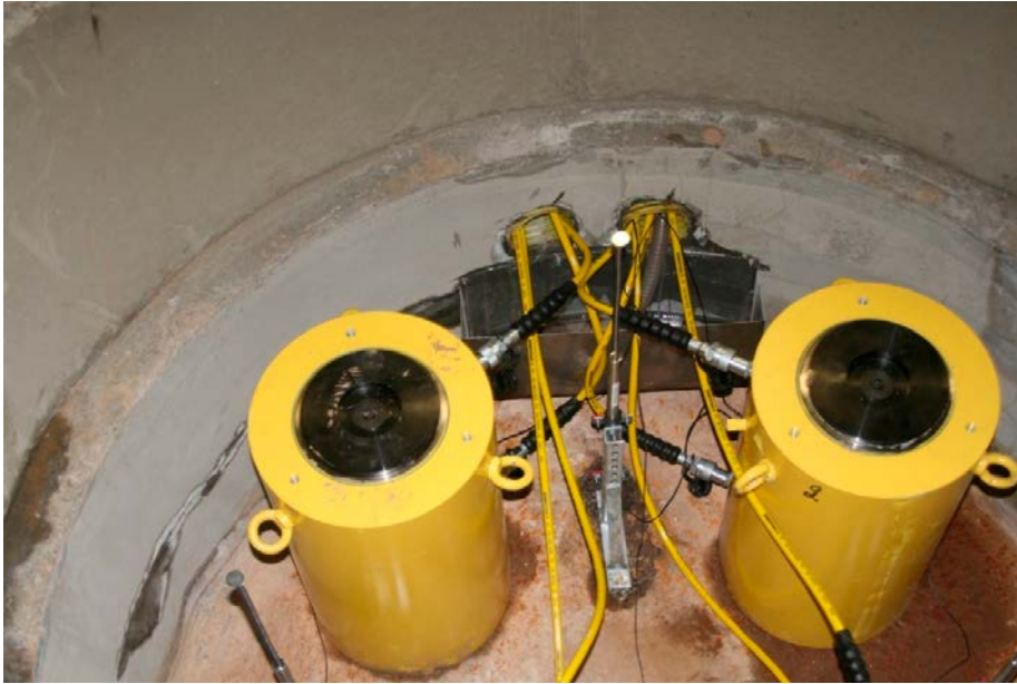
Figure 3-2. Close-up showing the entrance leading out cables from the deposition hole. Note the vessel that collects water leaking in from the cable ditch. A tube, connected to a pump, was continuously leading out water from the vessel.
