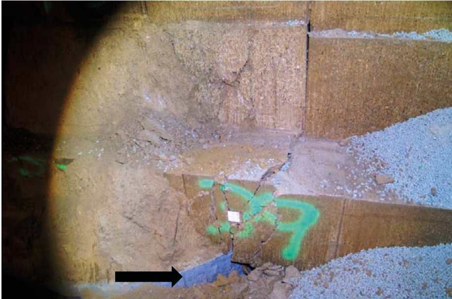
Figure 4-14. The edge of the buffer block (black arrow) and the sheared block above.
