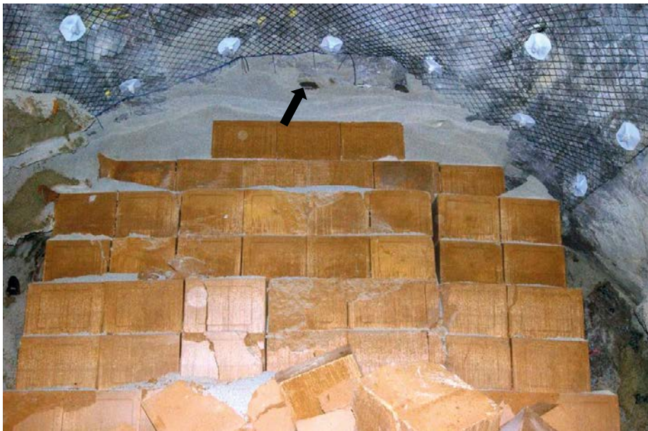
Figure 4-9. Photo showing the block stack top and the pressure sensor on the rock ceiling just above the deposition hole (black arrow).
