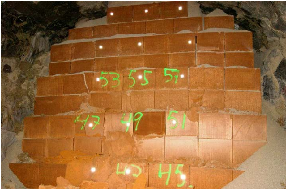
Figure 4-13. The vertical layer 4 (see Figure 3-10) above the deposition hole, where blocks were equipped with reflectors and their position determined with a total station before and after test.
