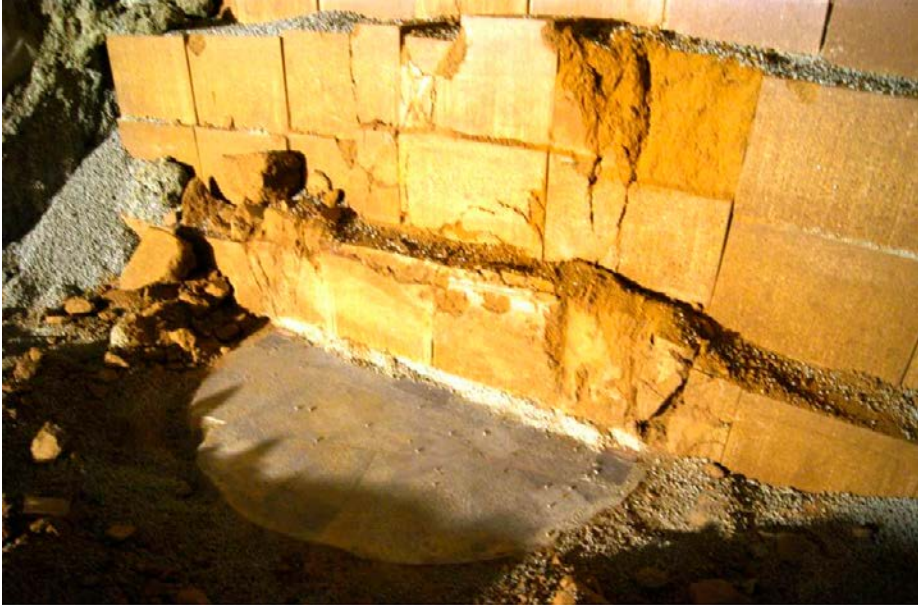
Figure 4-20. Photo showing the buffer block surface, the pellet layer and the backfill blocks at the midpoint of the deposition hole.
