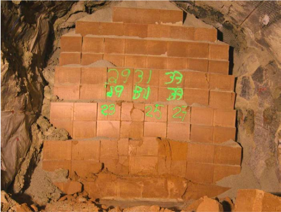
Figure 4-21. The backfill at the innermost part of the deposition hole in vertical layer 2 (see Figure 3-10). The shear and fracture surfaces can be seen very clearly.
