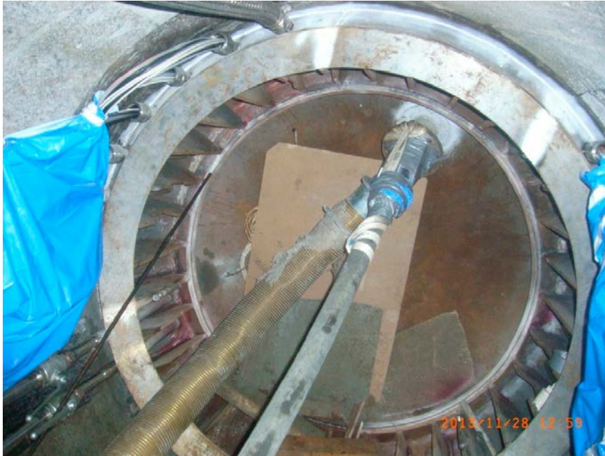
Figure 9-14. T-connector connected to the pellets filling hole in the plug.
