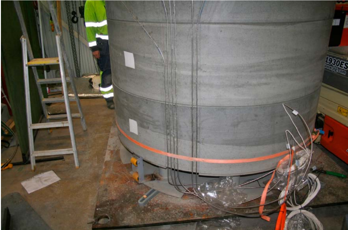
Figure 8-4. Lower part of one of the composite components, with the cable piping milled into and running along its periphery to the cable block. The pipes and cable rolls were later secured inside the cable block.
