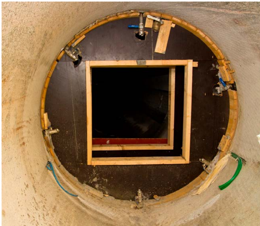
Figure 5-4. Form-work for the casting of the fastening ring.
