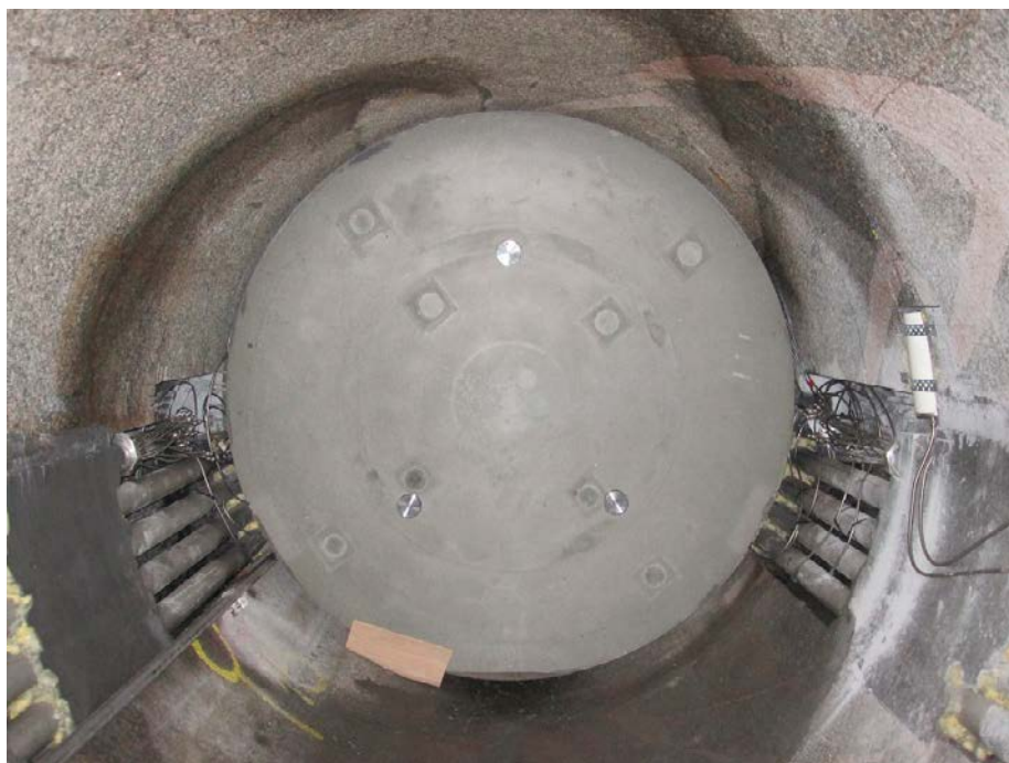
Figure 9-8. Outer distance block deposited.
