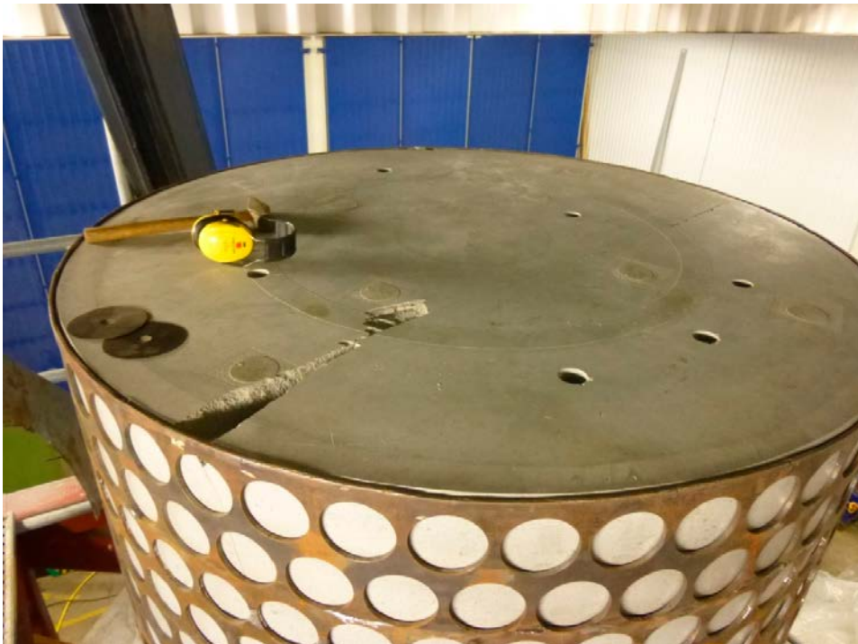
Figure 8-9. Top block placed inside the Supercontainer. The three pieces could be lifted individually by the mechanical lifting tool and positioned with tight fit, like a jigsaw puzzle. Machining of the height of the final ring ensured a total buffer height corresponding well with the height of the shell.
