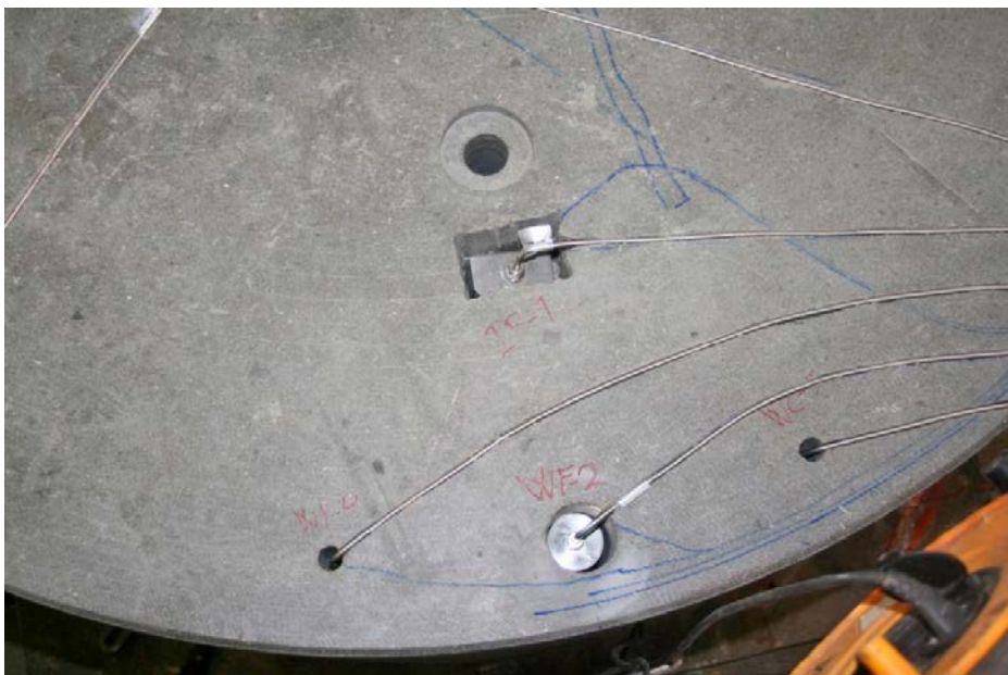
Figure 8-3. Sensors in place and ready for filling of bentonite powder around and on top of them. The hole in the upper part of the picture is one of the holes for the segmented lengthwise rods.
