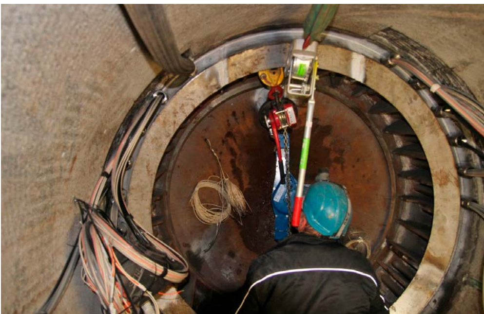
Figure 9-12. Raising of the cap by use of chain pulleys.
