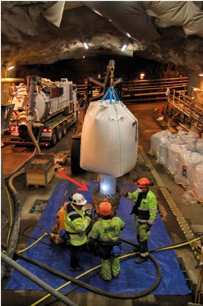
Figure 9-13. Pellets blower (red arrow) placed immediately outside the drift with pellets being filled. In the background, to the left, is the sewage truck used to suck out air and dust from the compartment.
