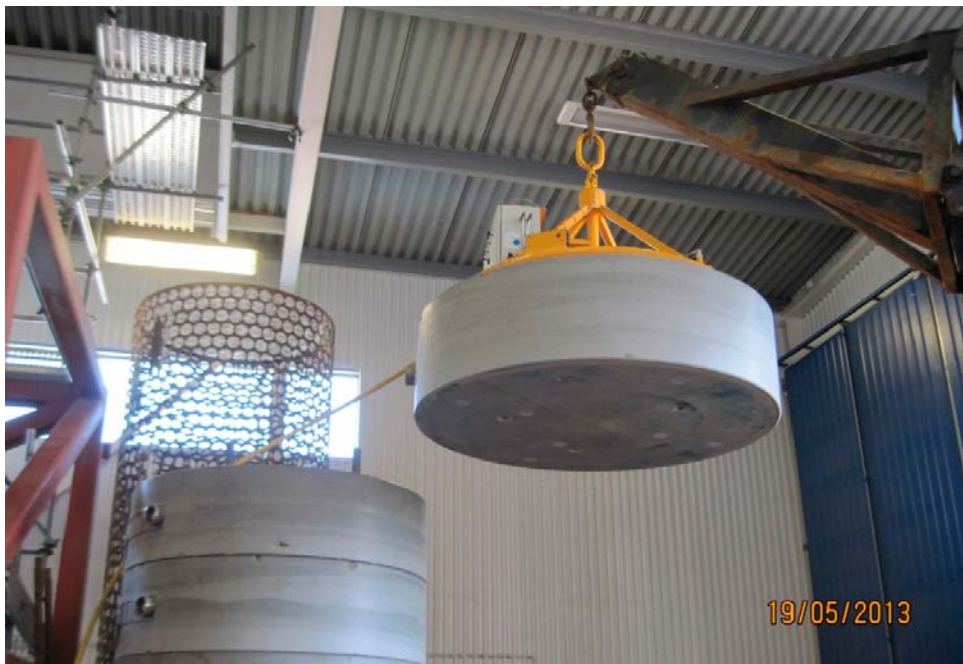
Figure 7-2. A Distance block segment being placed using a wheel loader and a vacuum tool in the controlled environment of the assembly facility. The distance block feet can be partially seen to the left on the stack of blocks.
