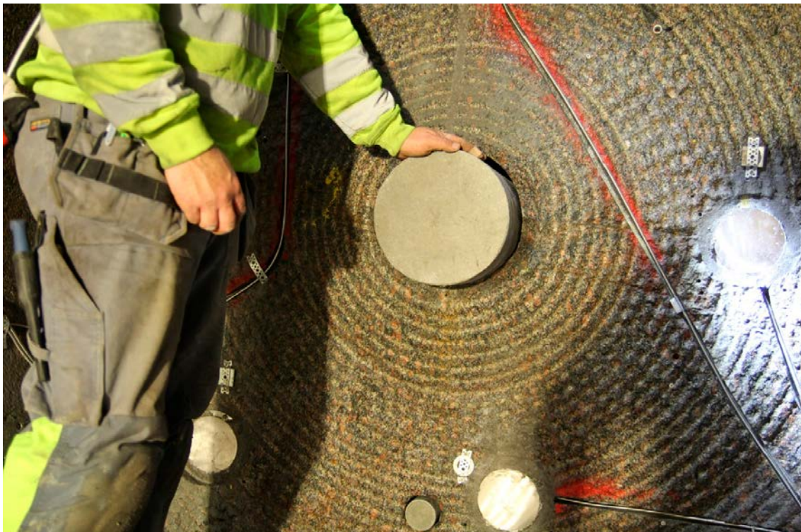
Figure 9-2. Bentonite filling components placed in the remainder of the main pilot hole, centre of picture, and in the 76 mm characterisation hole seen at the bottom of the picture. Also seen are three of the drift front total pressure sensor with their piping sawed into the rock and by their side a small distance placed to ensure that the first distance block would not crush them.
