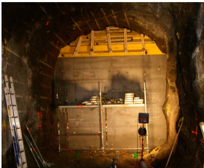
Figure 3-2. Concrete back-wall during the removal of the formwork.
