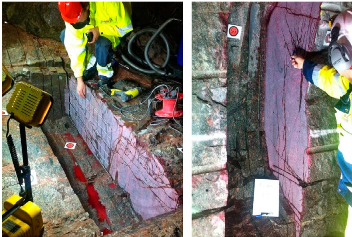
Figure 4-41. Mapping of blast induced fractures in TAS04 and TASN.
