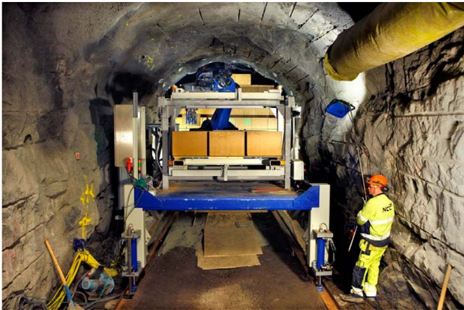
Figure 4-27. Robot platform with block feeding system and installation robot.
