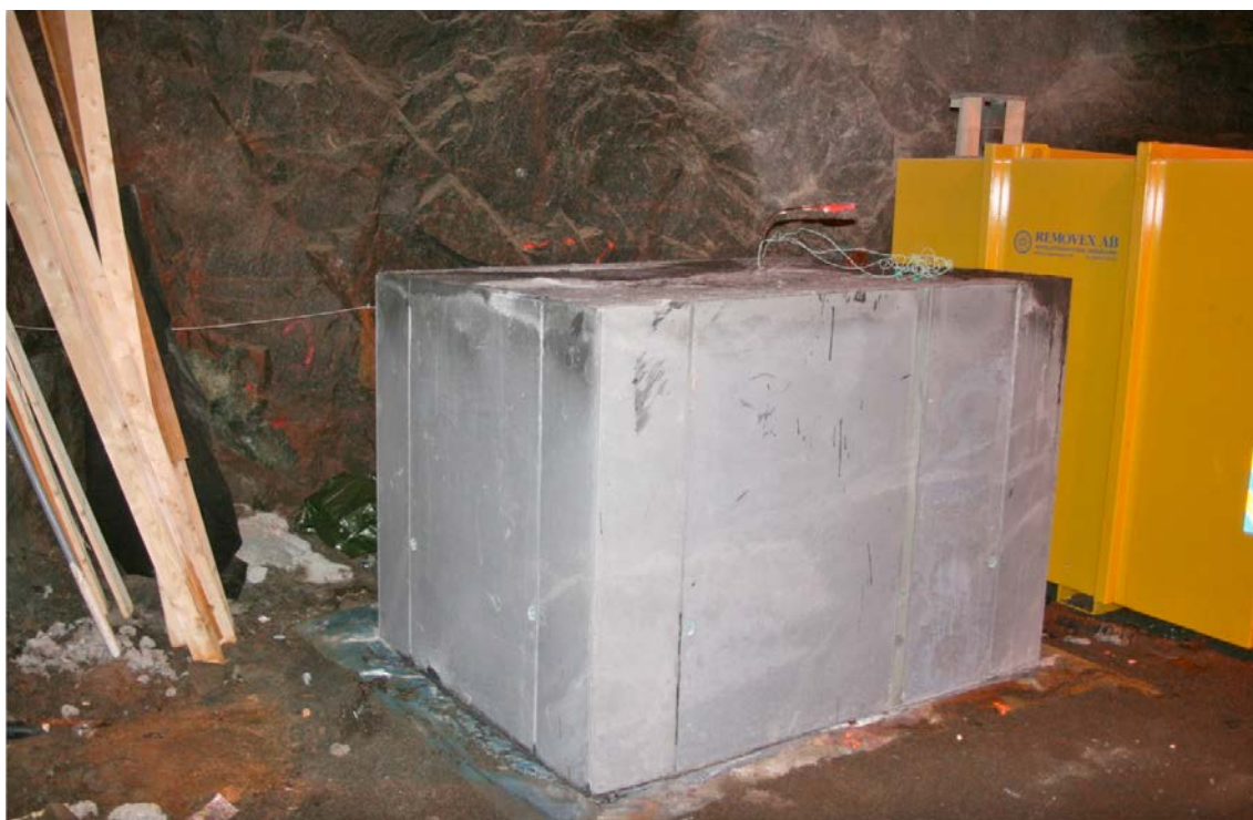
Figure 4-22. Monolite in low-pH concrete.
