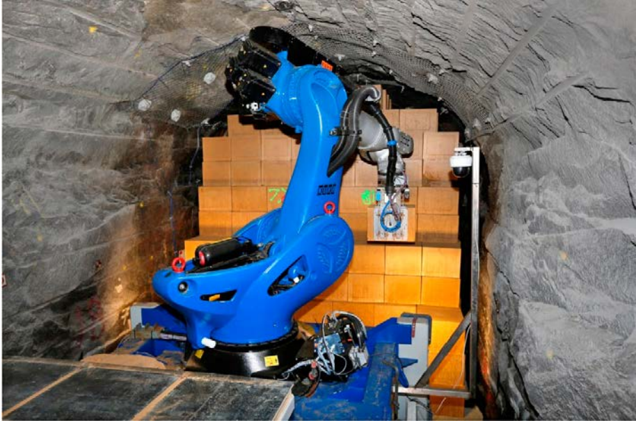
Figure 4-26. Installation robot operating in the TASS-tunnel.
