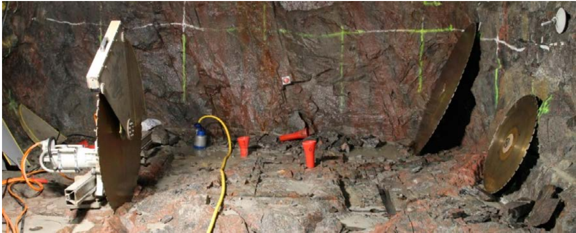
Figure 4-40. Ongoing sawing work in the floor of TAS04, section 34 m.
