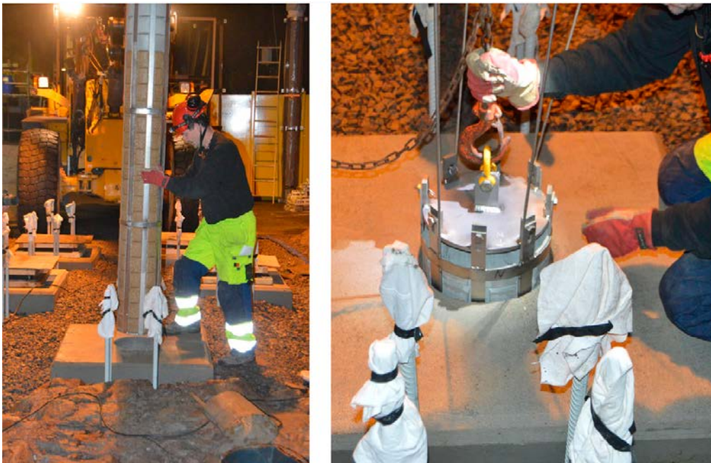
Figure 4-17. Lowering the bentonite package into the deposition hole.
