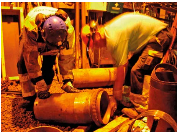
Figure 3-14. Drillers tightening the leading edge attached to the end of the capturing ring on the end of the core recovery barrel at ground level at the TRUE-1 drill site.
