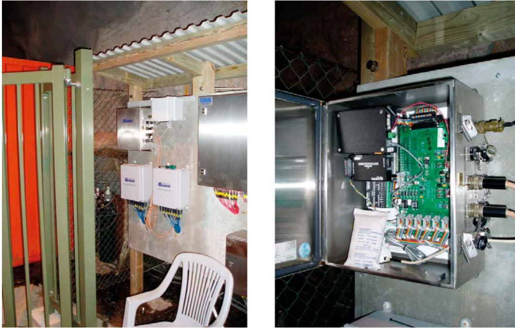
Figure 3-5. Data loggers for the hydromechanical equipment, located in Tunnel G.
