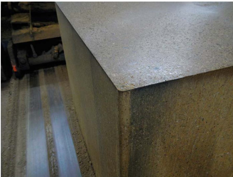
Figure 5-26. Close-up of one of the vertical edges.
