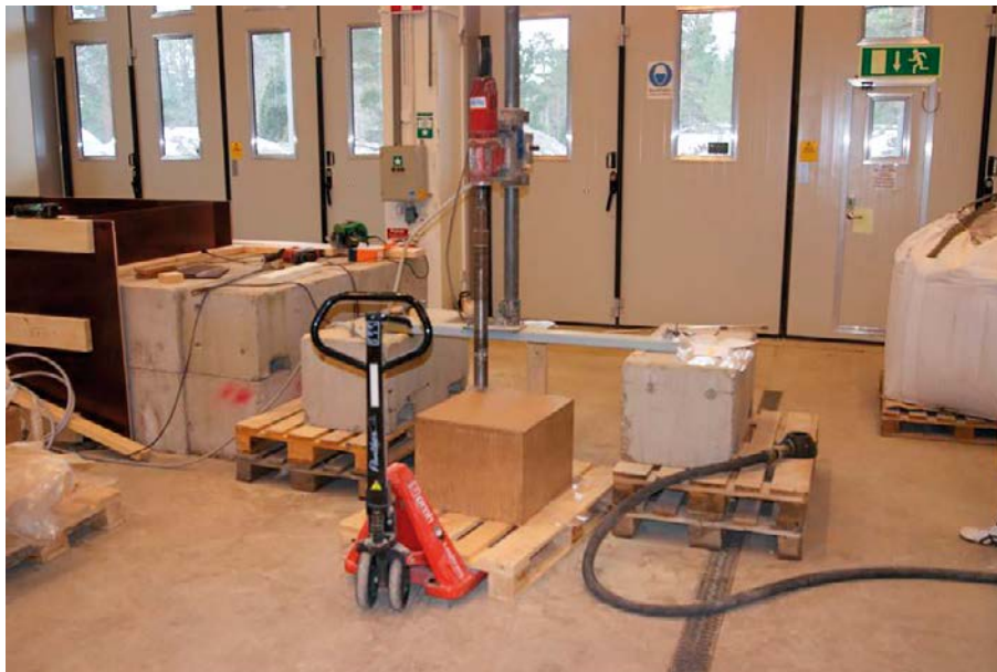
Figure 4-6. Photo showing the core drilling equipment used for the block sampling.
