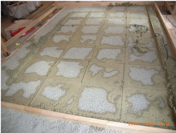
Figure 5-6. Photo taken after removal of the blocks. Water has entered mainly on the sides of the stack but also in the gaps between the blocks. (Johnsson 2011).
