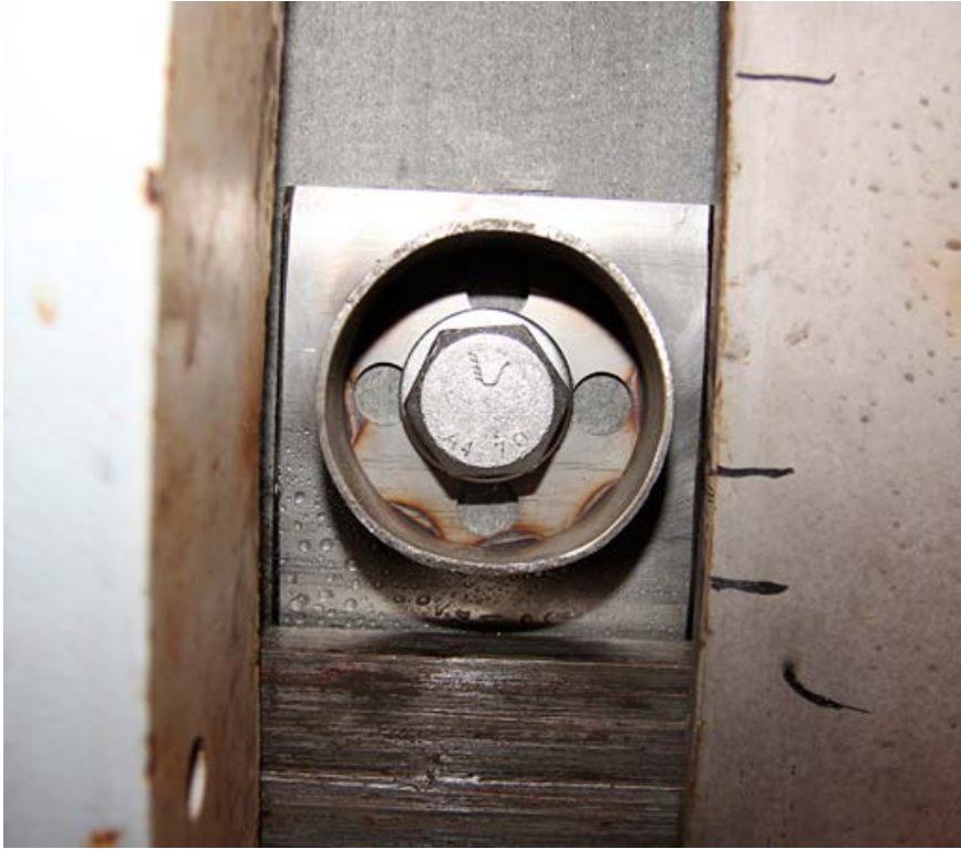
Figure 4-3. Slight deformation of the distance block foot after the deposition test. No cracking in the bentonite and firm fastening after the test.
