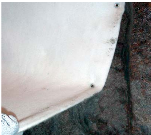
Figure 5-1. Testing the attachment by pulling the geotextile.
