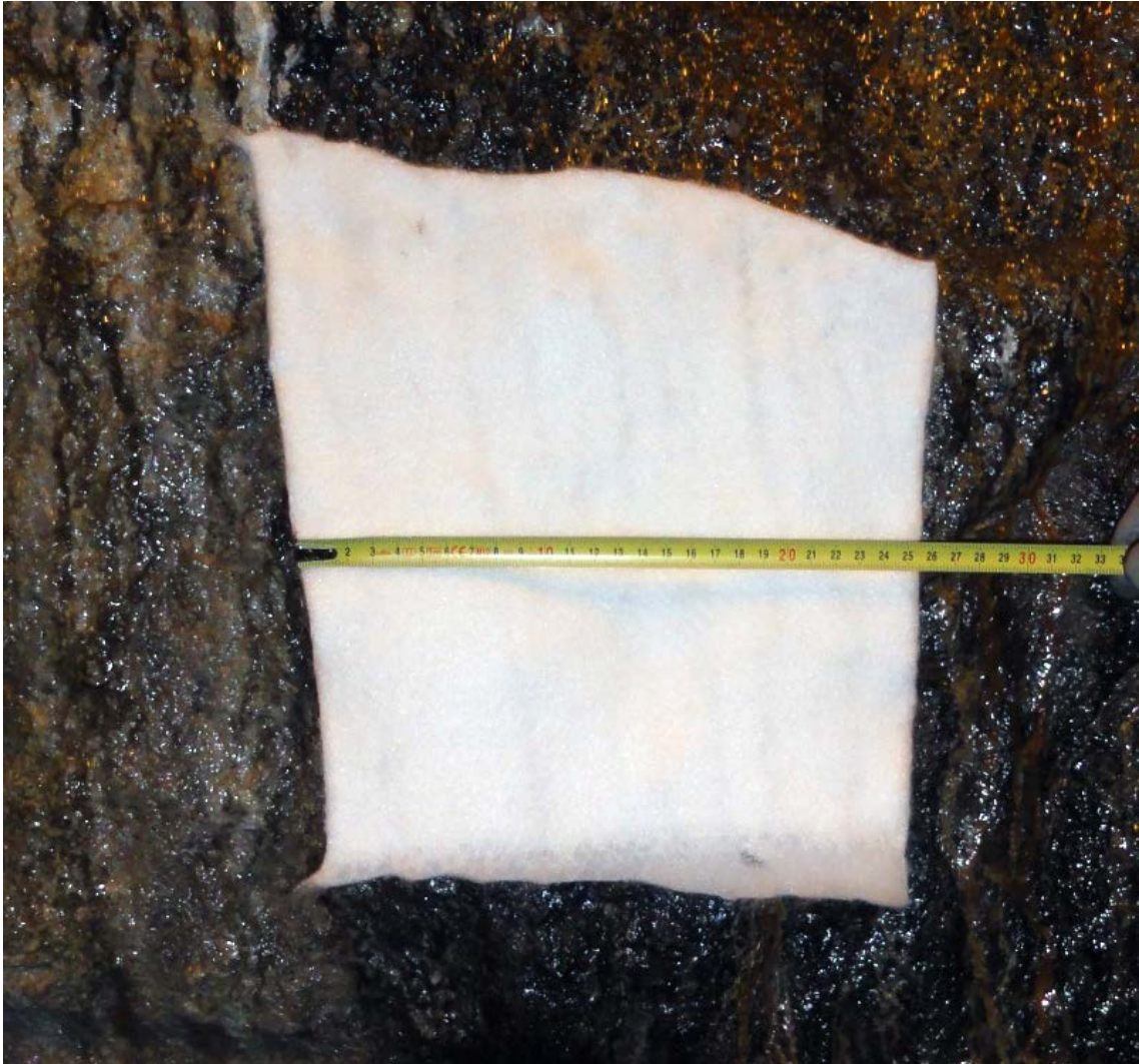
Figure 5-5. The small geotextile sections on the wall.
