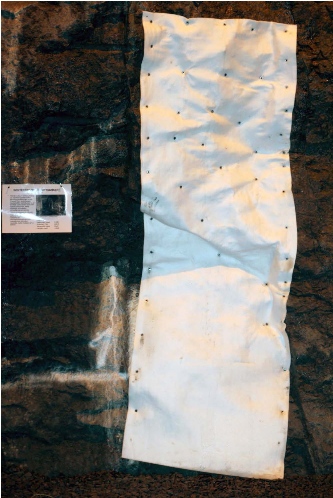
Figure 5-2. The attached geotextile.
