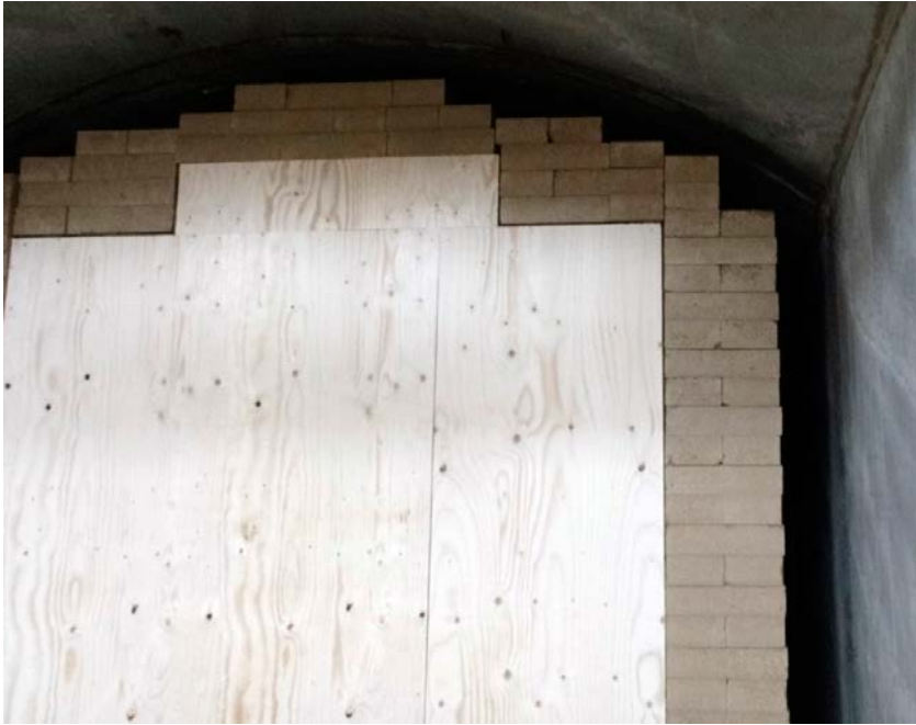
Figure 4-2. The backfill blocks, before the pellet installation.
