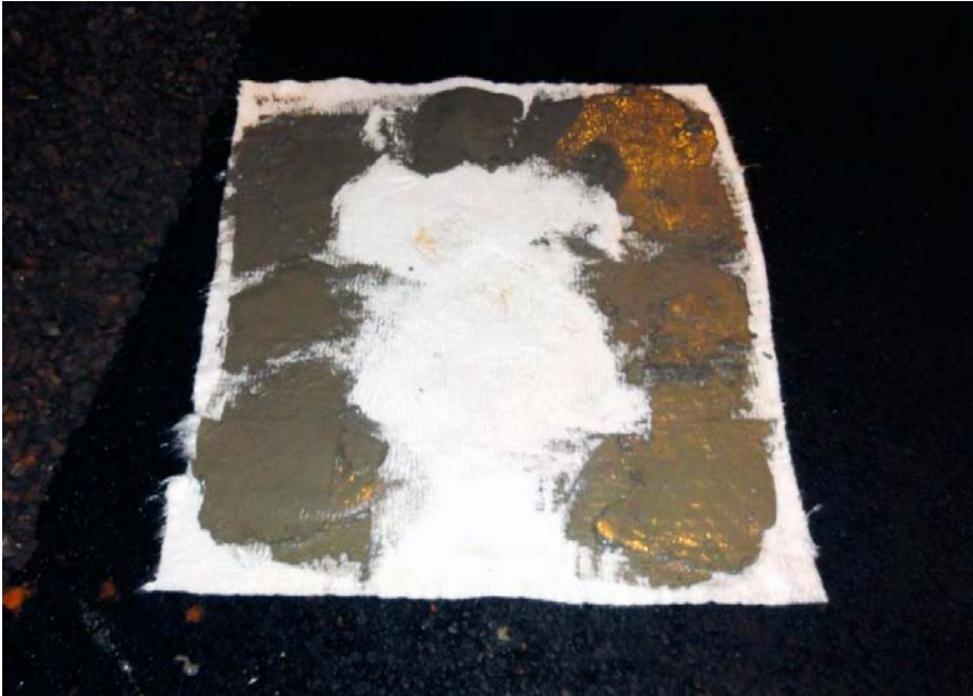
Figure 5-6. The glass fibre fabric with cement ready to be installed onto the rock surface.
