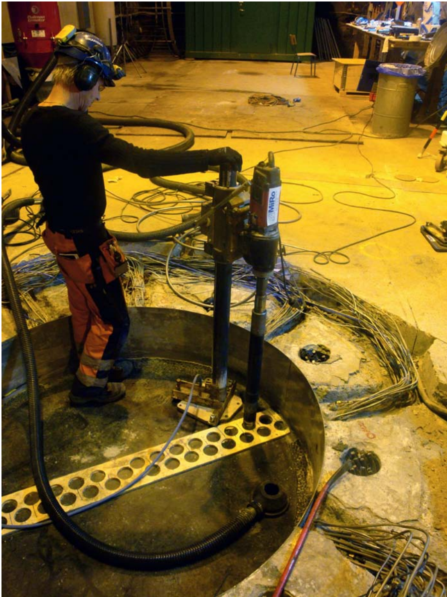
Figure 2-1. The drilling rig placed on top of block C4.
