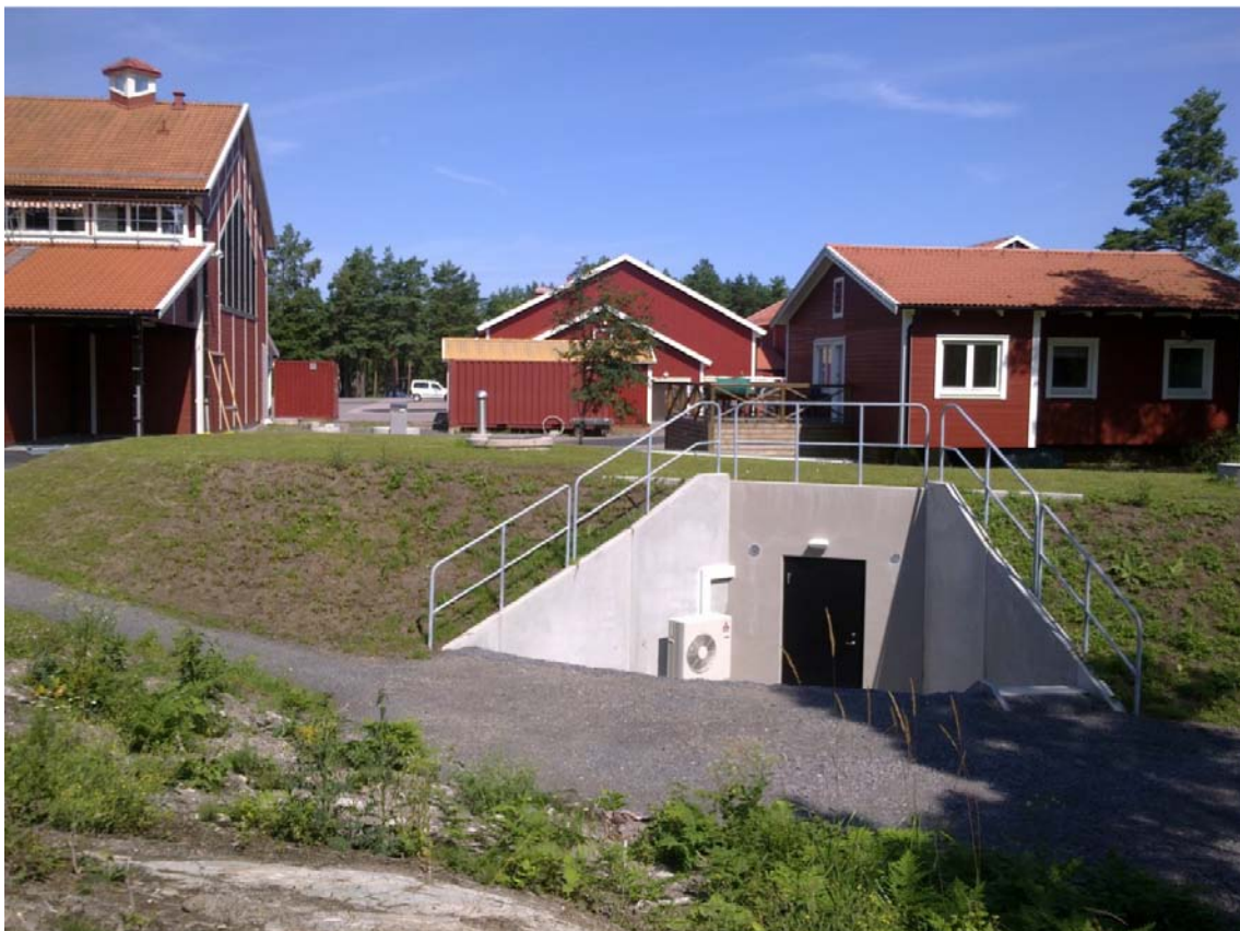
Figure 6-7. The new water and sewer construction allows to be pumped in a two-kilometre long pipeline to OKG's treatment plant.
