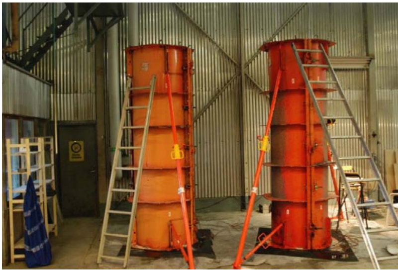
Figure 3-11. Two cylindrical steel moulds, diameter 0.85 m and height 3 m, instrumented with temperature gauges and one LVDT at the top to measure the settlement, were filled with low-pH SCC.
