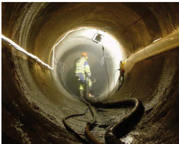
Figure 1-12. Photo of the Shotcrete Plug.
