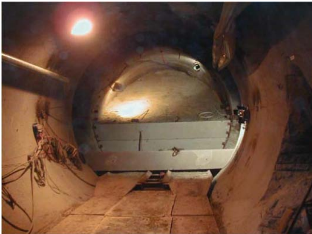
Figure 2-7. Assembly of the wall with prefabricated concrete beams.
