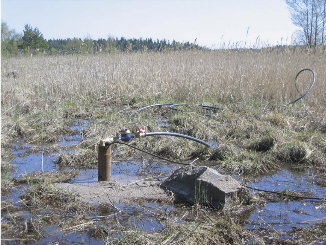
Figure 4-1. Pumping well SFM0074, flow meter, and hose for discharge of water from the well to Lake Bolundsfjärden.
