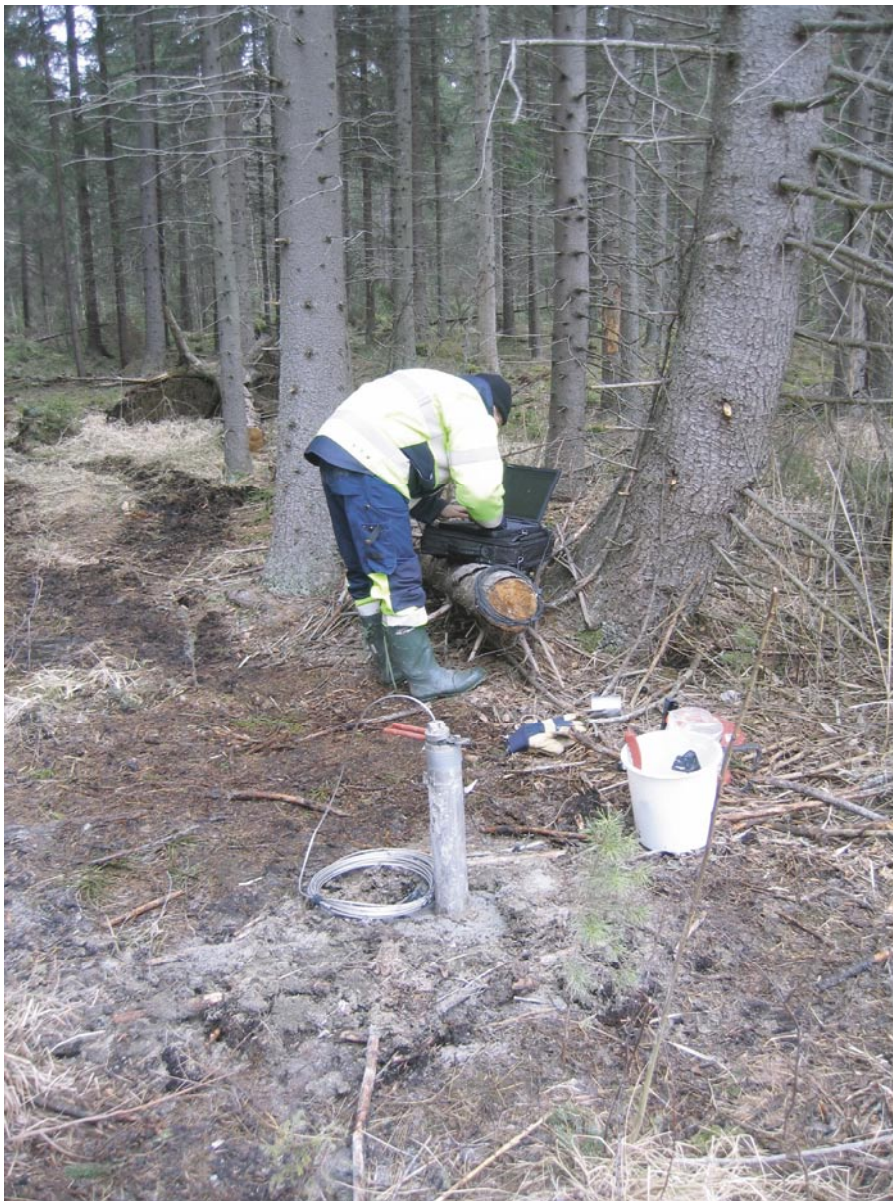
Figure 4-1. Groundwater monitoring well SFM0067. Cover pipe in stainless steel for protection of the HDPE stand pipe.
