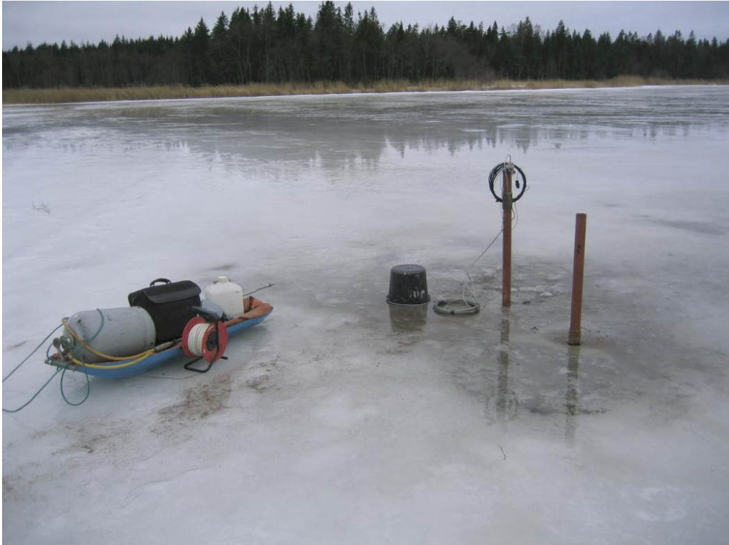
Figure 4-2. Groundwater monitoring well SFM0065 installed in soil below open water.
