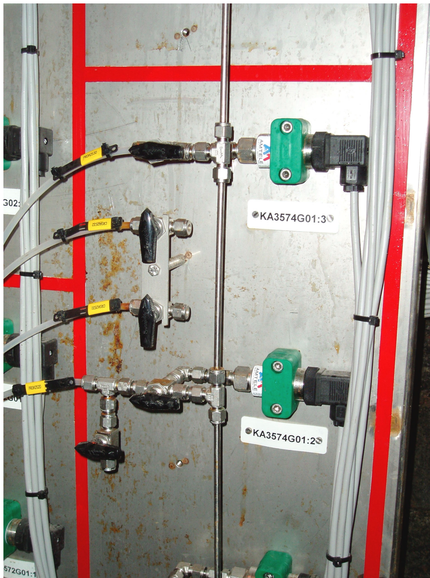
Figure 4-2 Pressure transducers connections
