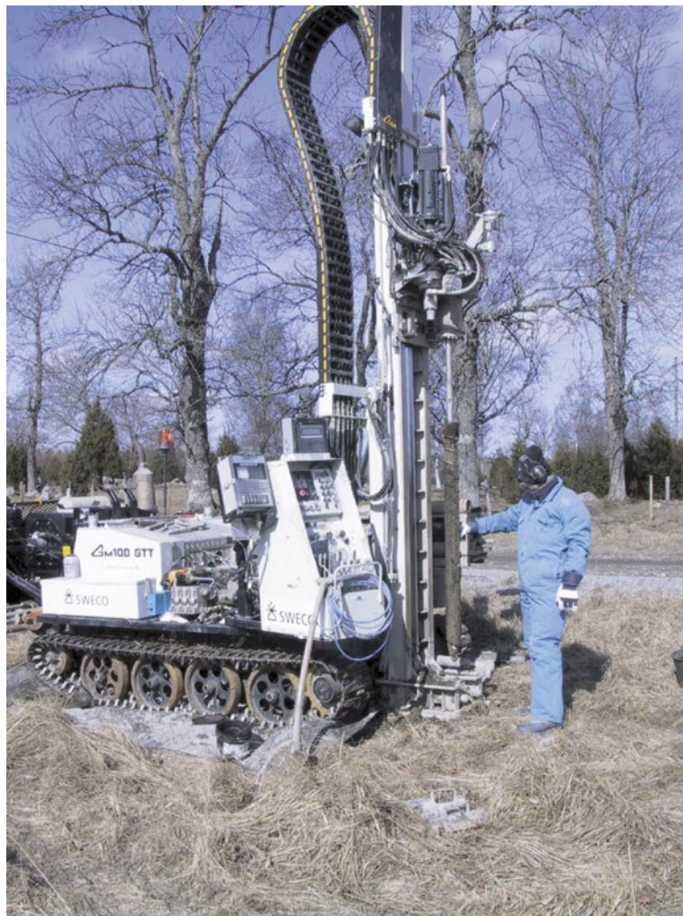
Figure 3-1. Drilling rig GeoMachine GM 100 GTT.
