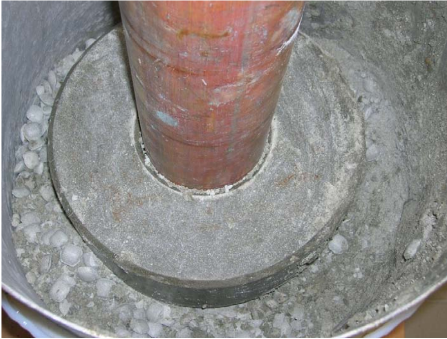
Figure A8-3. Photo taken during excavation. The pellets filling is only partly wetted. The blocks are almost unaffected of the water and major cracks can be seen.
