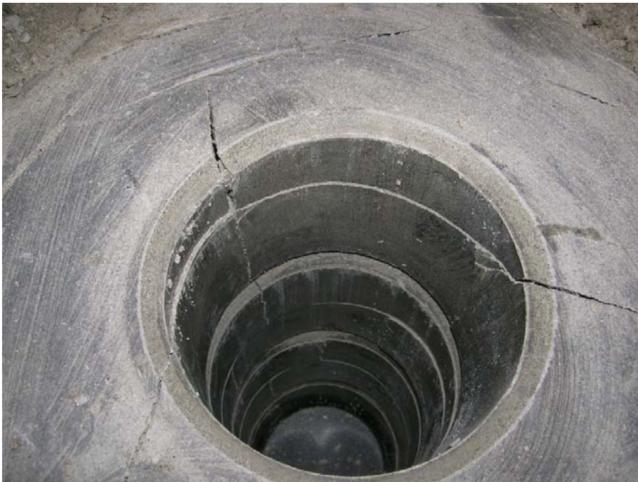
Figure A3-4. Photo taken during excavation. The large cracks in the blocks are very clear.
