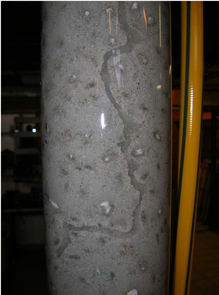
Figure 4-8. Photo showing a typical channel where all water is flowing.
