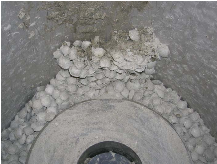
Figure A4-4. Photo taken during excavation. The water have been flowing from the inflow point up along the wall, only influencing a small part of the pellet filling.
