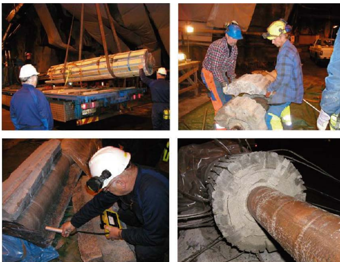
Figure 4-7. Upper left: Placement of the entire parcel on a lorry for transport to a dry niche. Upper right: Removal of the first piece of covering rock. Lower left: Radioactivity check of the uncovered bentonite in the lower part of the parcel. Lower right: Partly water unsaturated bentonite exposed during the sampling of the upper part of the parcel.
