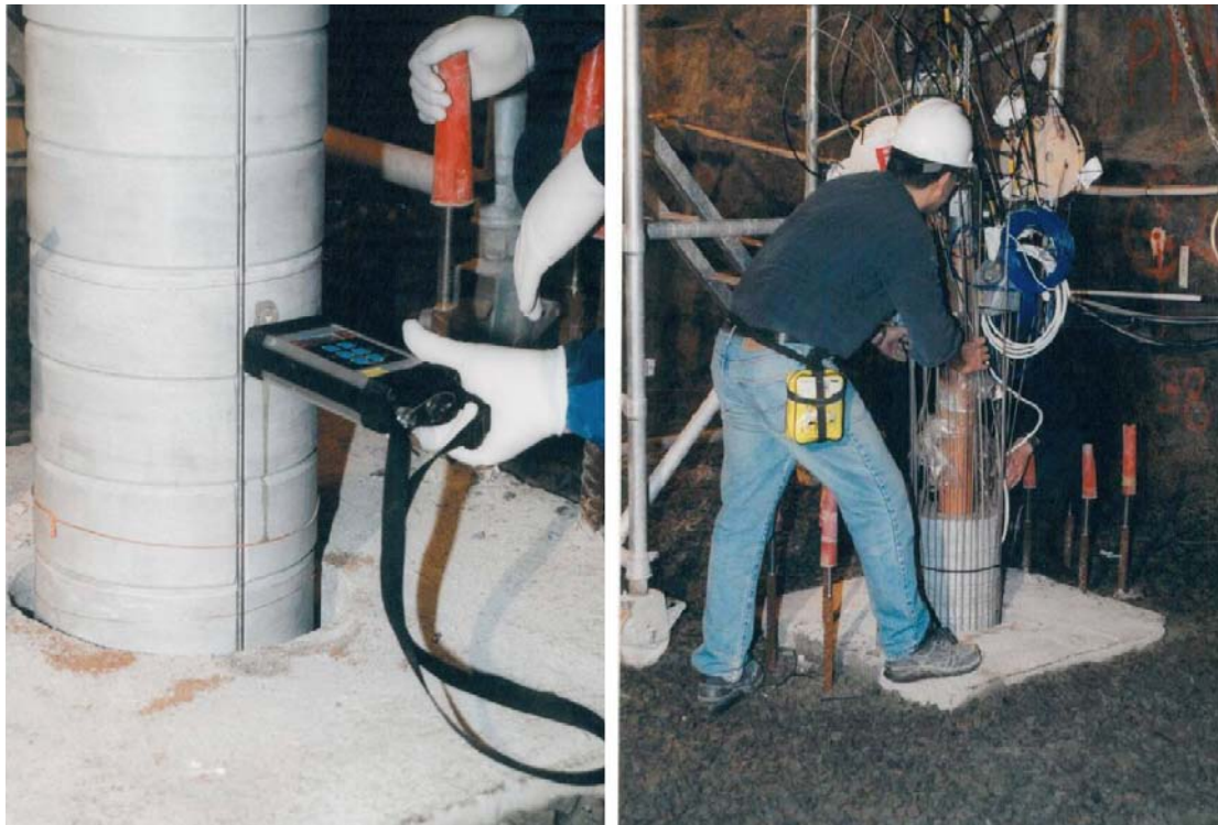
Figure 4-1. Example of activities during the lowering of the A0 parcel into the test hole. Left: Check of radiation from the radioactive tracer test plug in block no.5 during the initial lowering of the parcel. The wet spot is due to the small amount of water which was used to seal the test plug. Right: Only the 3 uppermost blocks (36 to 38) remain visible in the tunnel. Note the large number of cable containing tubes from the sensors on the outside of this upper part of the test parcel.
