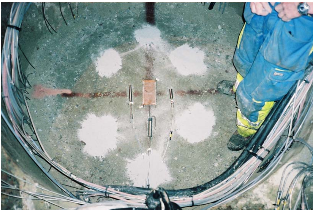
Figure 5-10. The backfilling and instrumentation of the top of a deposition hole.
