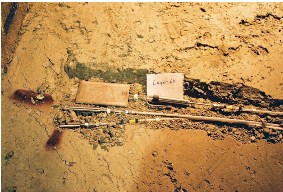
Figure 5-7. Installation of sensors in the backfill.
