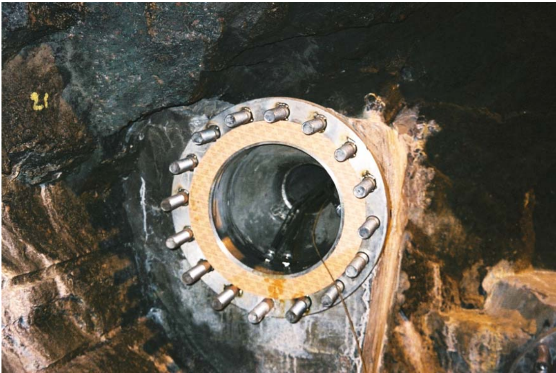
Figure 2-3. Photos showing the installation of steel tubes in the rock (upper) and one completed lead through installed in the rock (without steel flange and cables).
