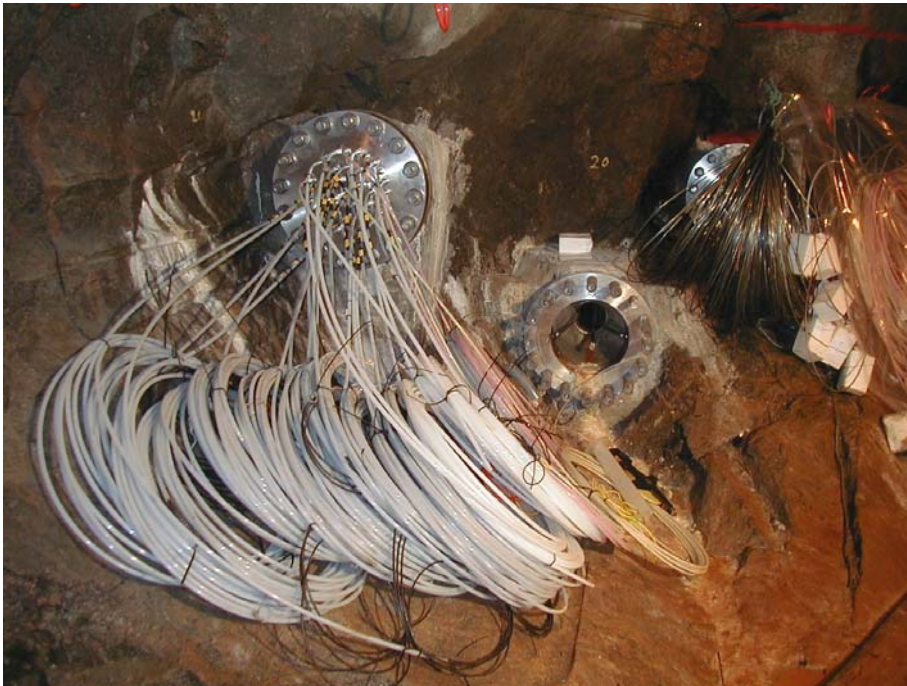
Figure 5-6. Cable package in place.
