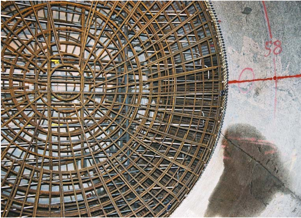
Figure 8-4. The outer reinforcement of the plug.
