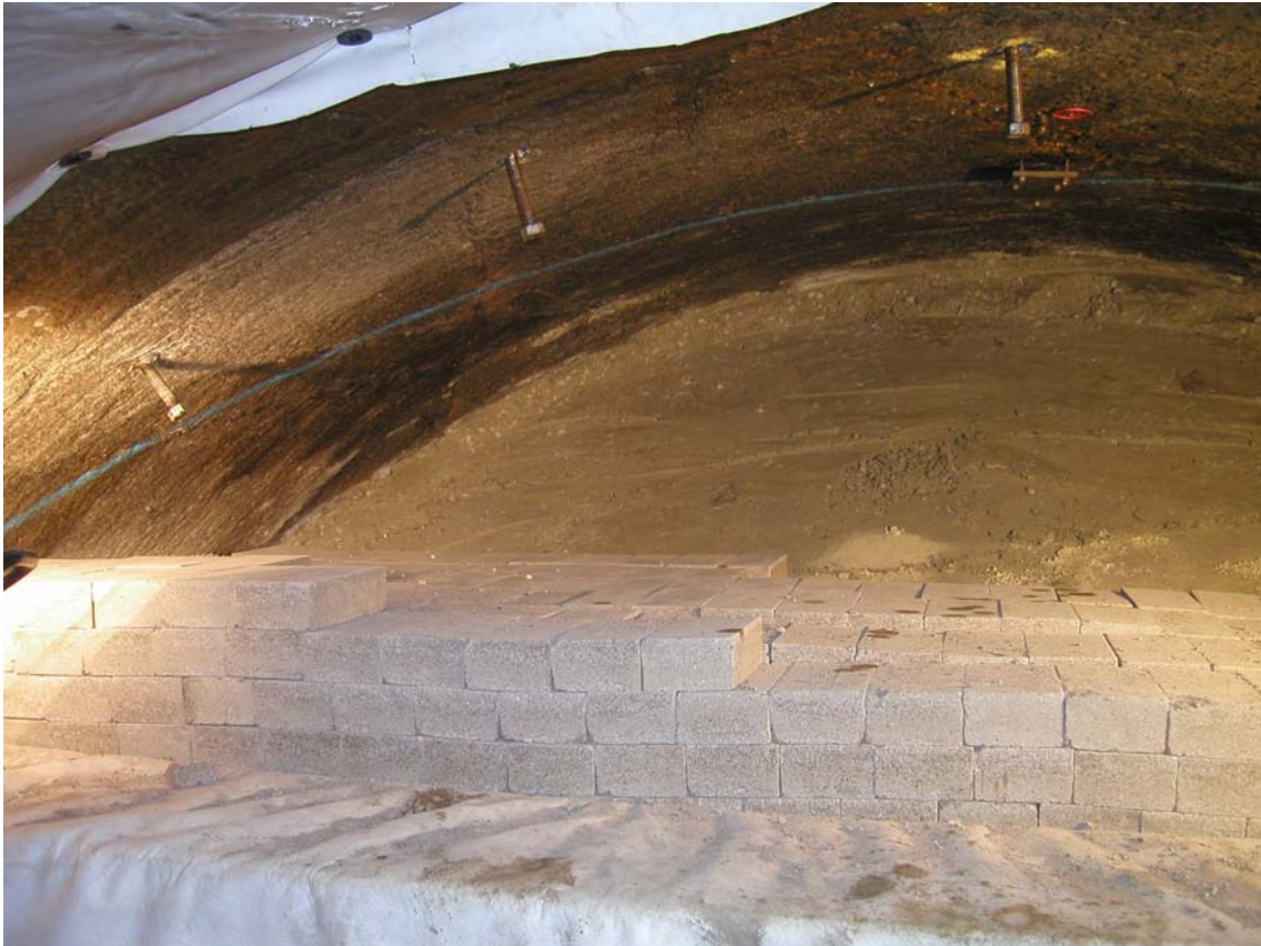
Figure 5-14. Placing blocks and pellets in the volume at the roof.
