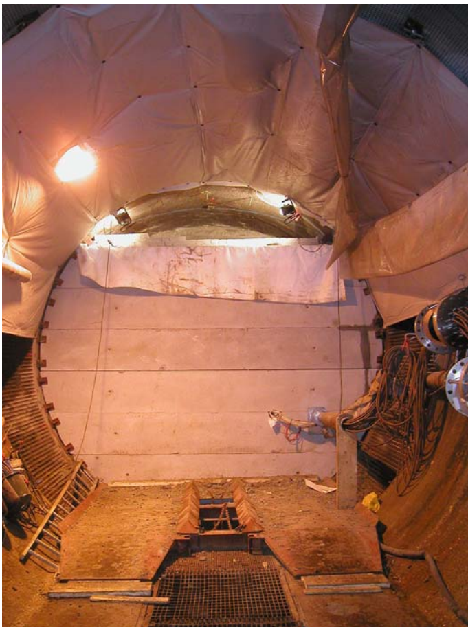
Figure 5-13. Installation of the concrete beams.
