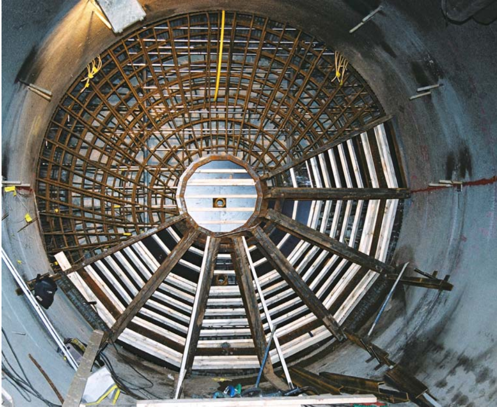
Figure 6-6. The reinforcement and part of the framework put in place.
