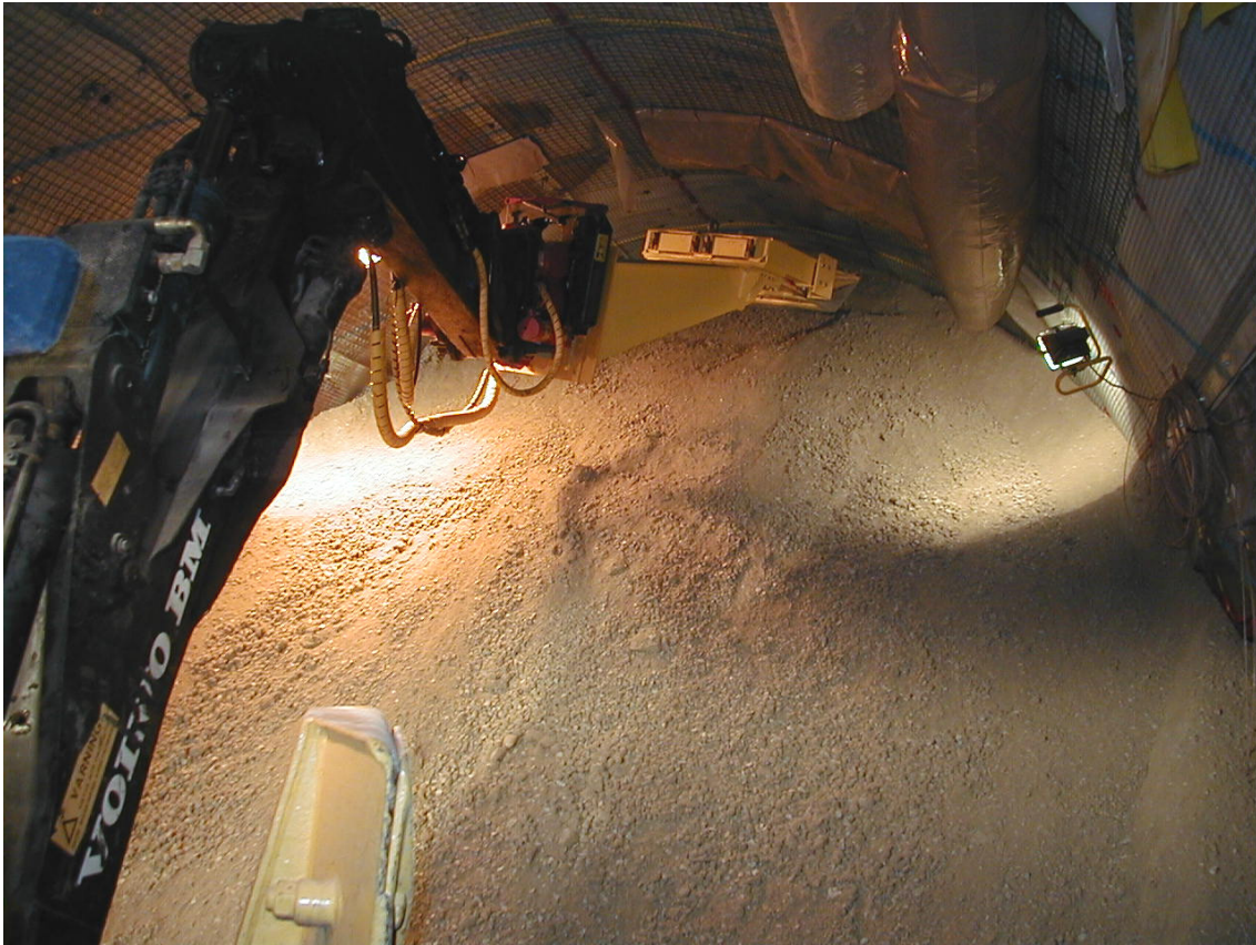
Figure 5-4. The roof compactor.
