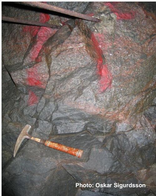
The TASA-tunnel, right wall, section 46-47 m. Boundary between the rock types Fine grained dioritoid (lower part) and Ävrö granodiorite (upper part) (left). A 3D-model of the TASS-tunnel, section 3-20.7 m. The irregular black lines in the model show fractures, rock boundaries etc. (right).
