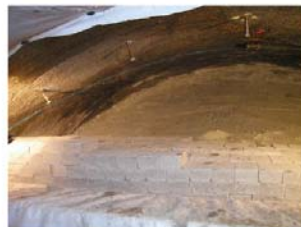
(b) Installation of blocks and pellets
