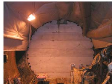
(c) Retaining wall before construction of concrete dome
