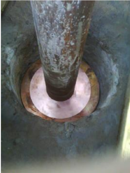
Installation of a copper plug in a 200 mm borehole.
