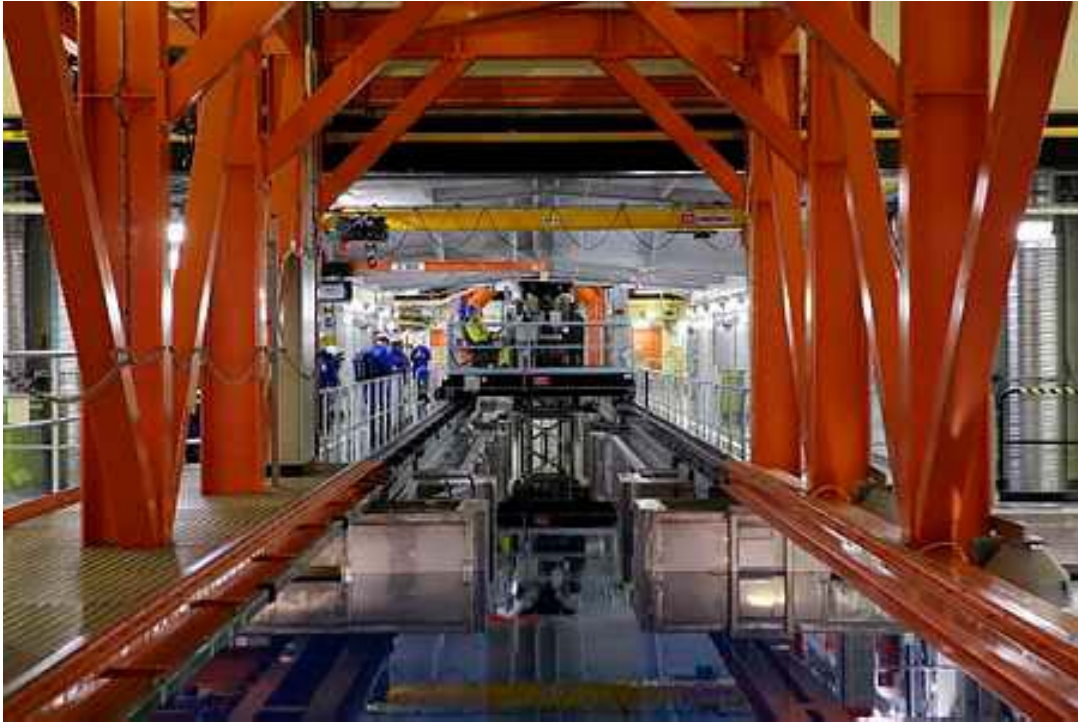
Figure 3-13. Clab is an example of a facility for wet storage of spent nuclear fuel.
