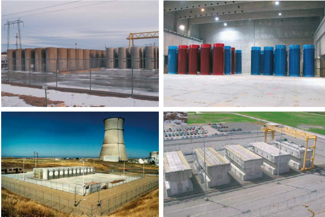
Figure 3-14. Examples of facilities for dry storage. At top left: outdoor storage of thick-walled cylindrical steel containers at Point Lepreau Generating Station (Source: NBPower Nuclear). At top right: CASTOR® containers (thick-walled cylindrical containers of cast iron) in storage building at Gorleben, Germany (Source: IAEA). At bottom left: outdoor storage in NUHOMS® (leaktight steel containers) at Susquehanna nuclear power plant in the USA (Source: IAEA). At bottom right: outdoor storage in CANSTOR® (tight metal containers surrounded by a concrete structure) at Gentilly-2 in Canada (Source: Hydro Quebec).
