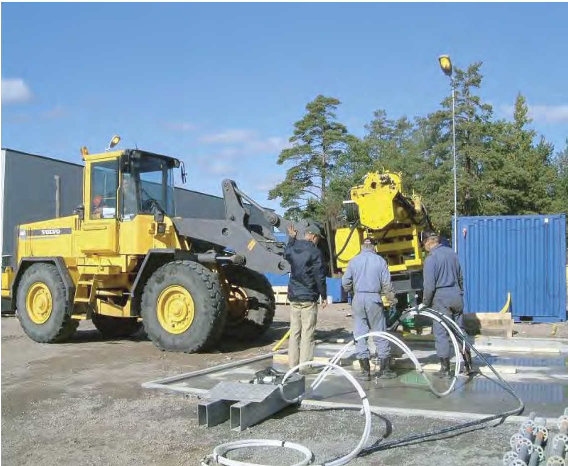
Figure 5-1. Drill site preparations.
