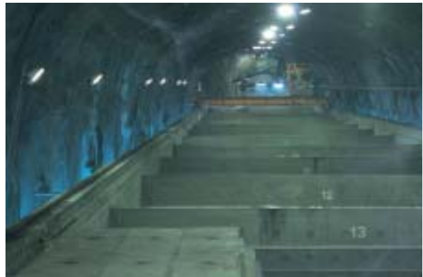
Rock vault for ILW.
