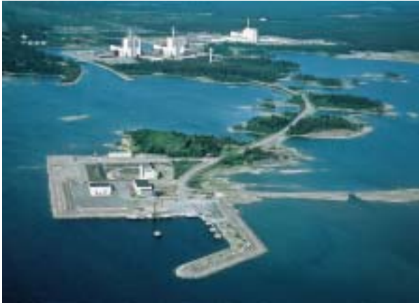
View of the above-ground complex.
